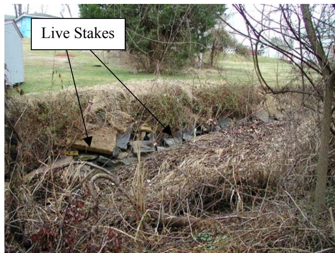
Figure 5.9: Live Stakes at Station 21+0
