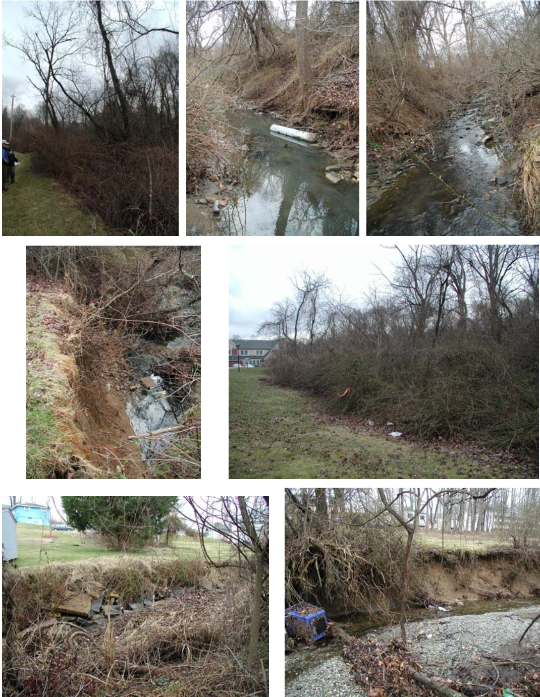
Clockwise from top left: Station 14+0-removal of multiflora rose by hand cutting and reforestation, Station 16+0- wing deflectors, Station 17+0-wing deflectors, Station 19+0-removal of multiflora rose by herbicide and reforestation, Station 23+0-root wads, Station 21+0- live stakes, and Station 18+0-coconut fiber roll and bank shaping
