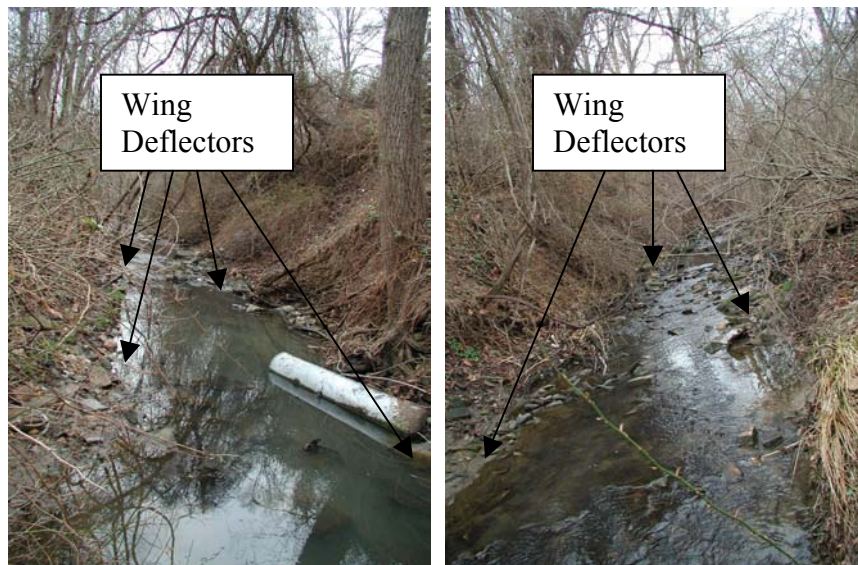
Figure 5.3: Wing Deflectors at Stations 16+0 and 17+0
