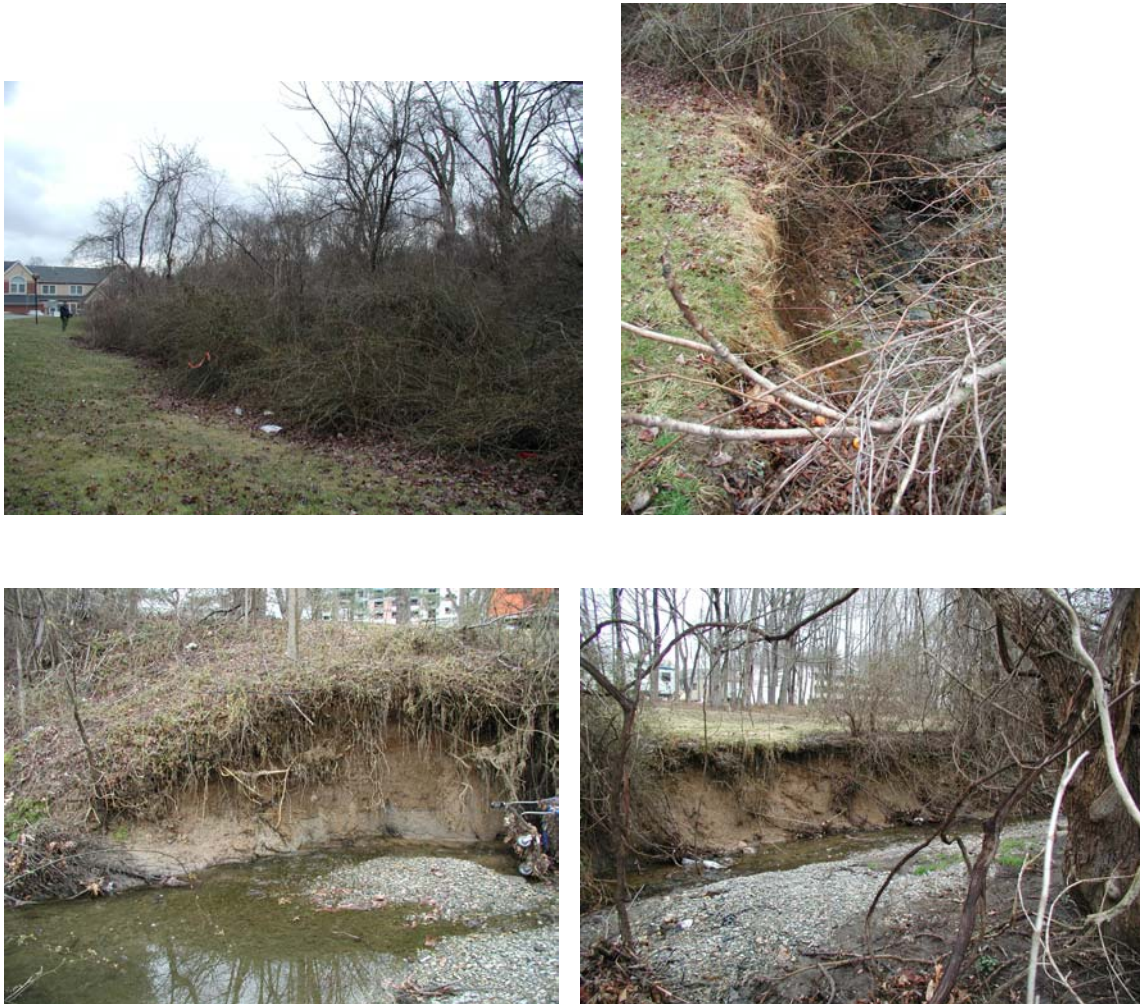
Clockwise from top left: multiflora rose along stream bank (14+0), vertical bank (18+0), erosion with litter from dormitories (23+0), longer look at extensiveness of the erosion (23+0).
