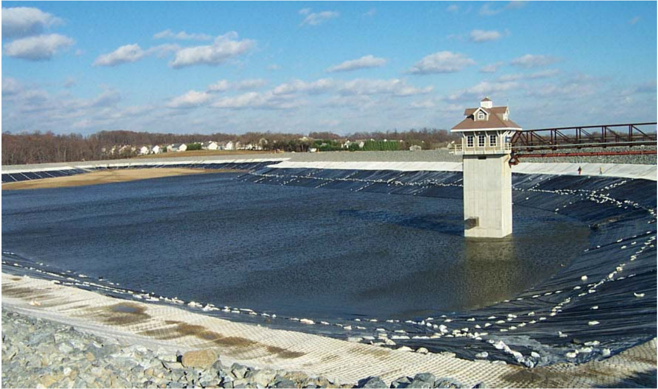
Newark Reservoir, looking northeast, December 2005.
