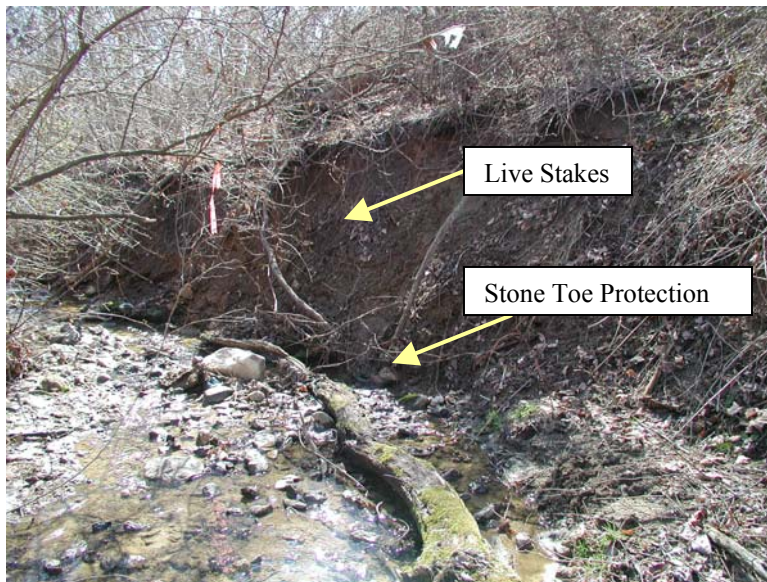
Figure 5.9: Location of Stone Toe Protection and Live Stakes
