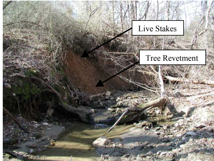
Figure 5.7: Location of Tree Revetment and Live Stakes
