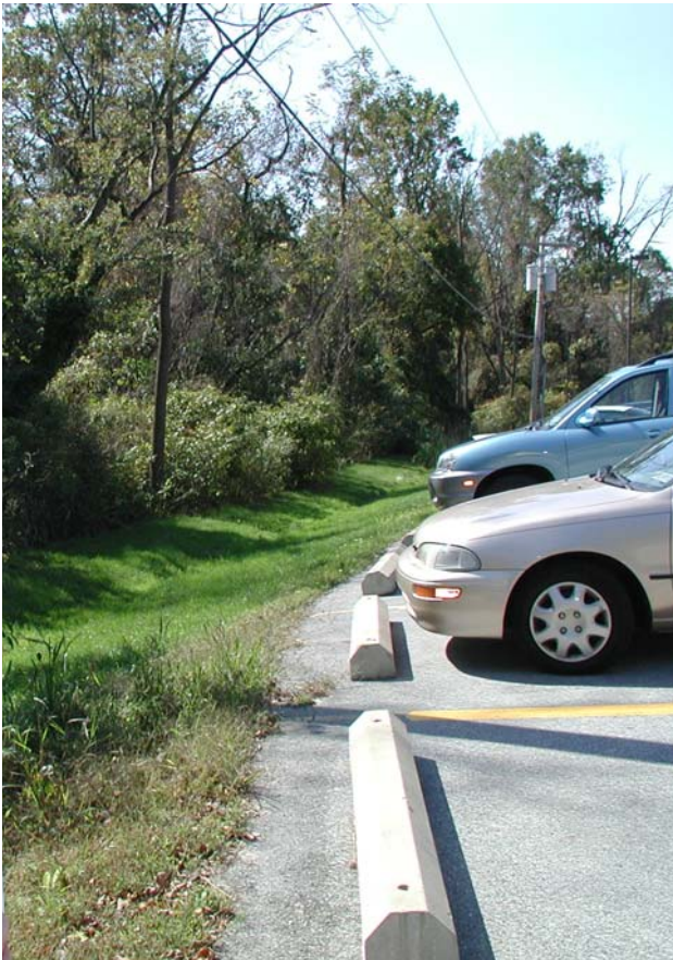
Figure 6: Image of Clayton Hall Stormwater Swale Running along the Alpha Sigma Alpha Parking Lot.
