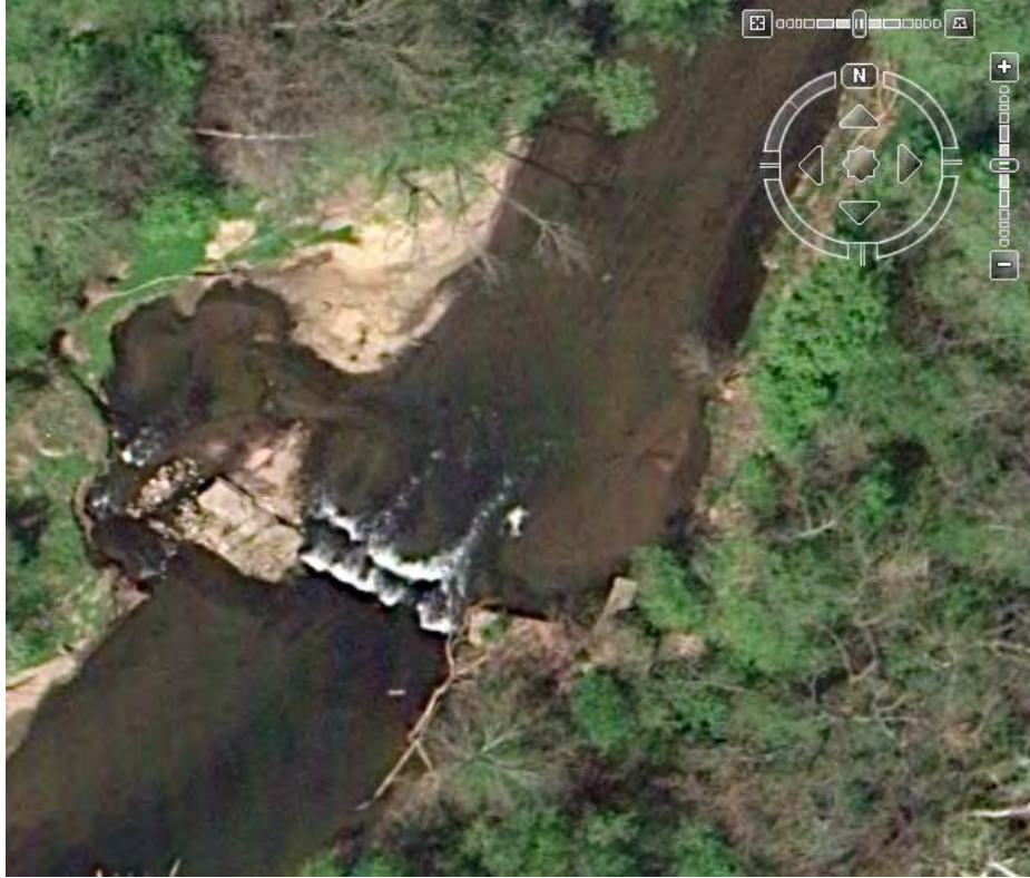
Plan view of White Clay Creek Dam No. 1. Note breach along overbank to left.
