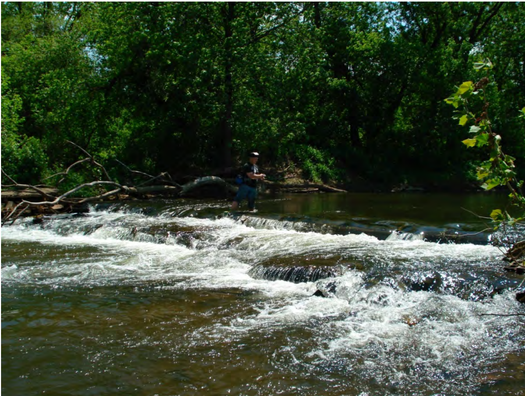
Dam No. 1 along the White Clay Creek (RM 4.2) at Delaware Park looking upstream
