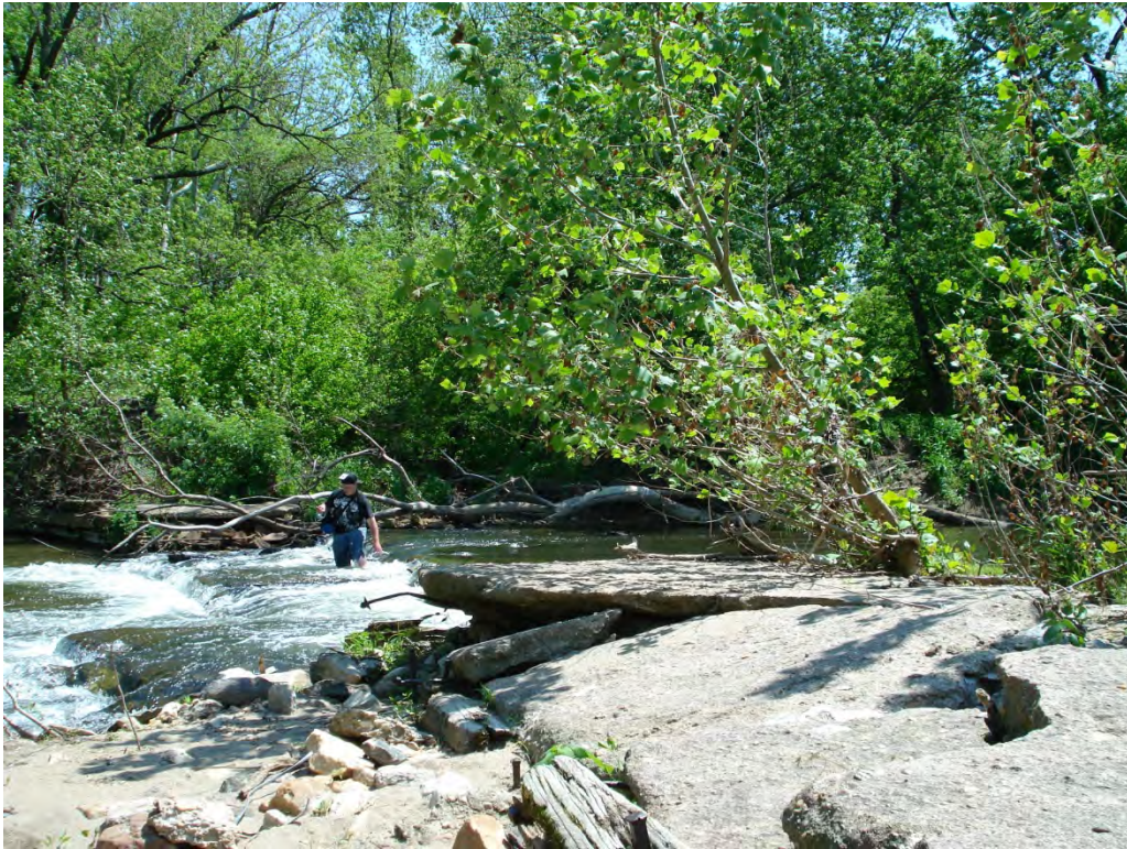
Dam No. 1 along White Clay Creek at Delaware Park looking toward left bank.
