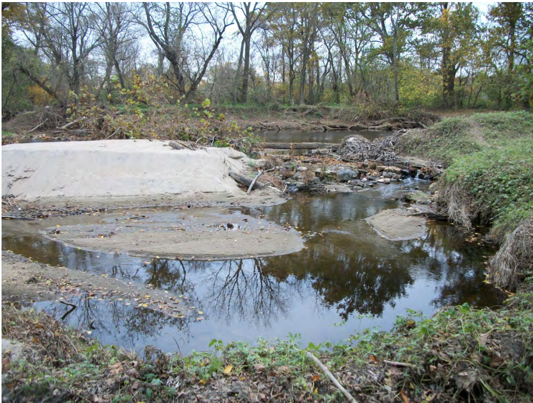
Looking upstream at Dam No. 1 (April 2011).
