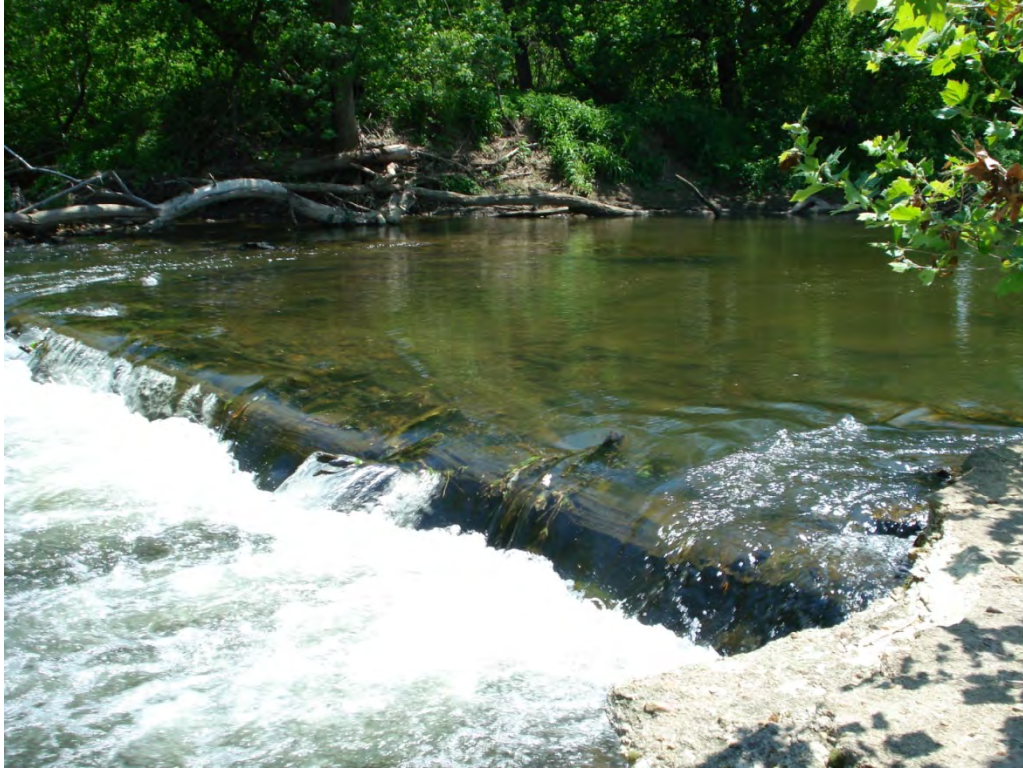
Dam No. 1 along White Clay Creek (RM 4.2) at Delaware Park, note timber frame
