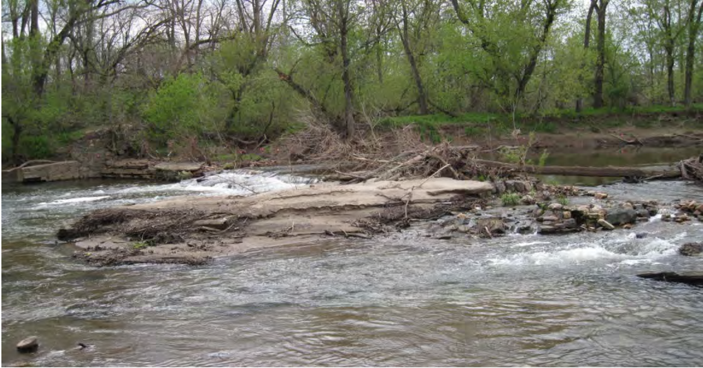
Dam No. 1 looking upstream (April 2011).
