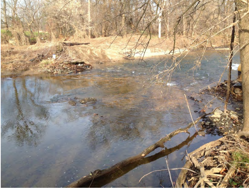
Removal of White Clay Creek Dam No. 1 (December 2014)
