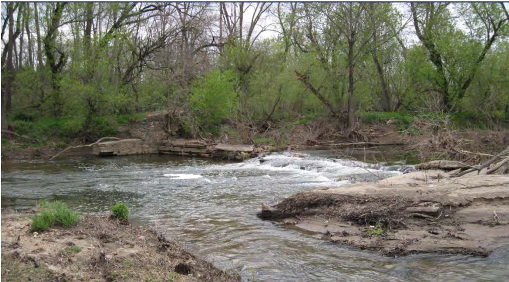
Dam No. 1 looking upstream (April 2011).
