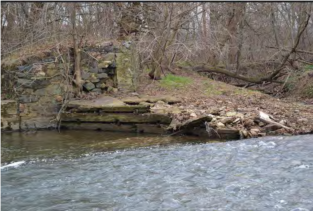
Historic timber crib to remain at White Clay Creek Dam No. 1 (December 2014)
