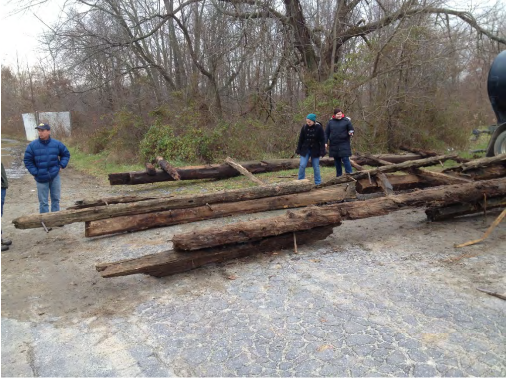
Timber remnants from White Clay Creek Dam No. 1 (December 2014)
