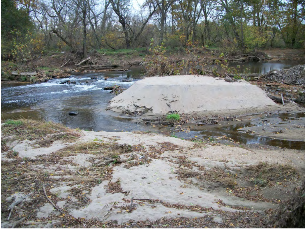
Looking south at Dam No. 1 (April 2011).
