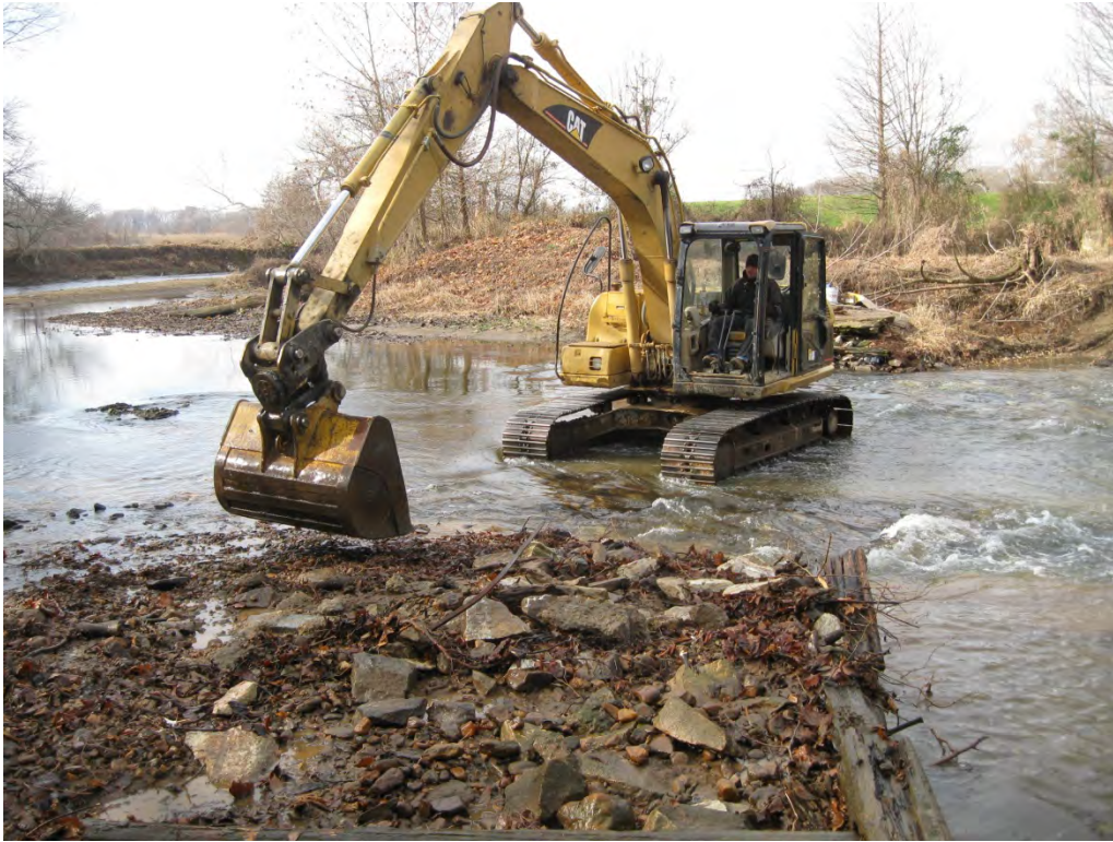
White Clay Creek Dam Removal (December 2014)
