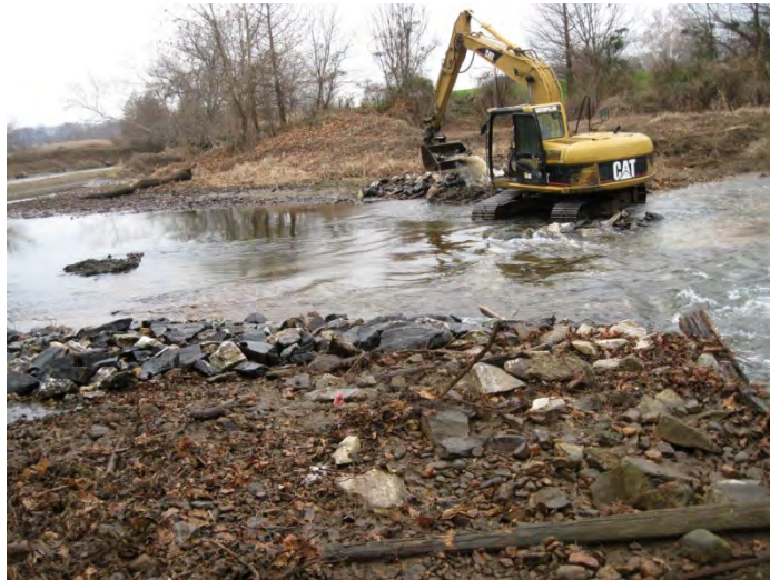
Figure 8. Removal of White Clay Creek Dam No. 1 in December 2015
