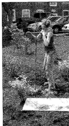
FIGURE 11. Performing soil borings to install pea gravel drains through clay layer.
