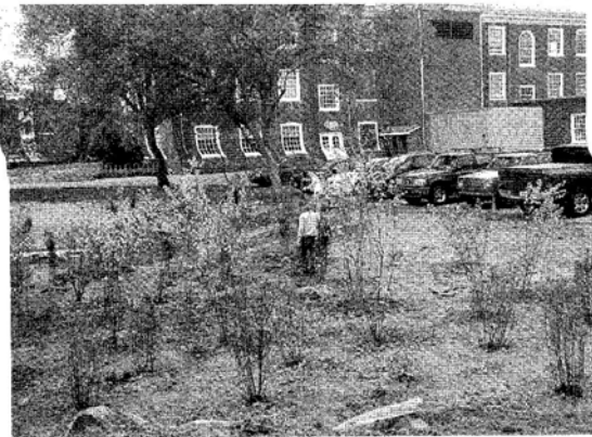
FIGURE 8. Installing the native plants at the University of Delaware rain garden.
