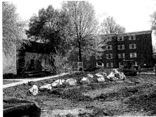
FIGURE 6. Earthwork and excavation at the University of Delaware rain garden.
