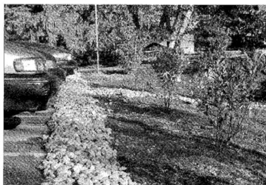
FIGURE 10. Installation of cobble erosion control filter strip.
