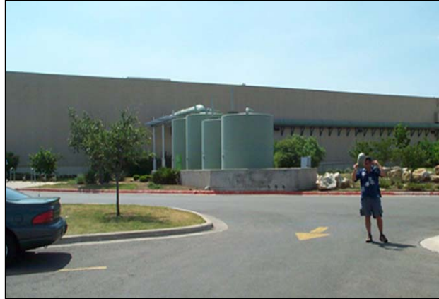
Figure 1b: Large Building Cistern System, Austin, TX
