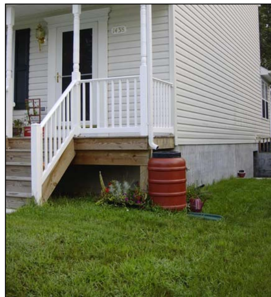
Figure 1: Installed Rain Barrel
