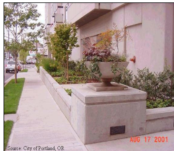
Figure 1: Portland Stormwater Planter
