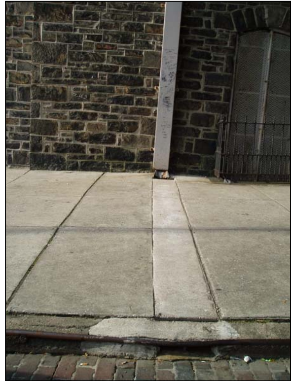
Figure 1: Downspout from St. Martin Church on Fayette.
