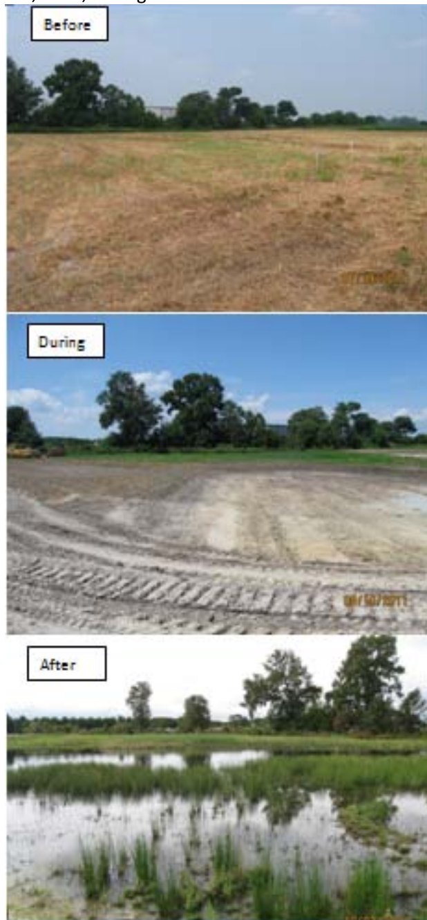
Figure 4. Example of wetland restoration BMP implemented by the Middle Chester River Partnership.
