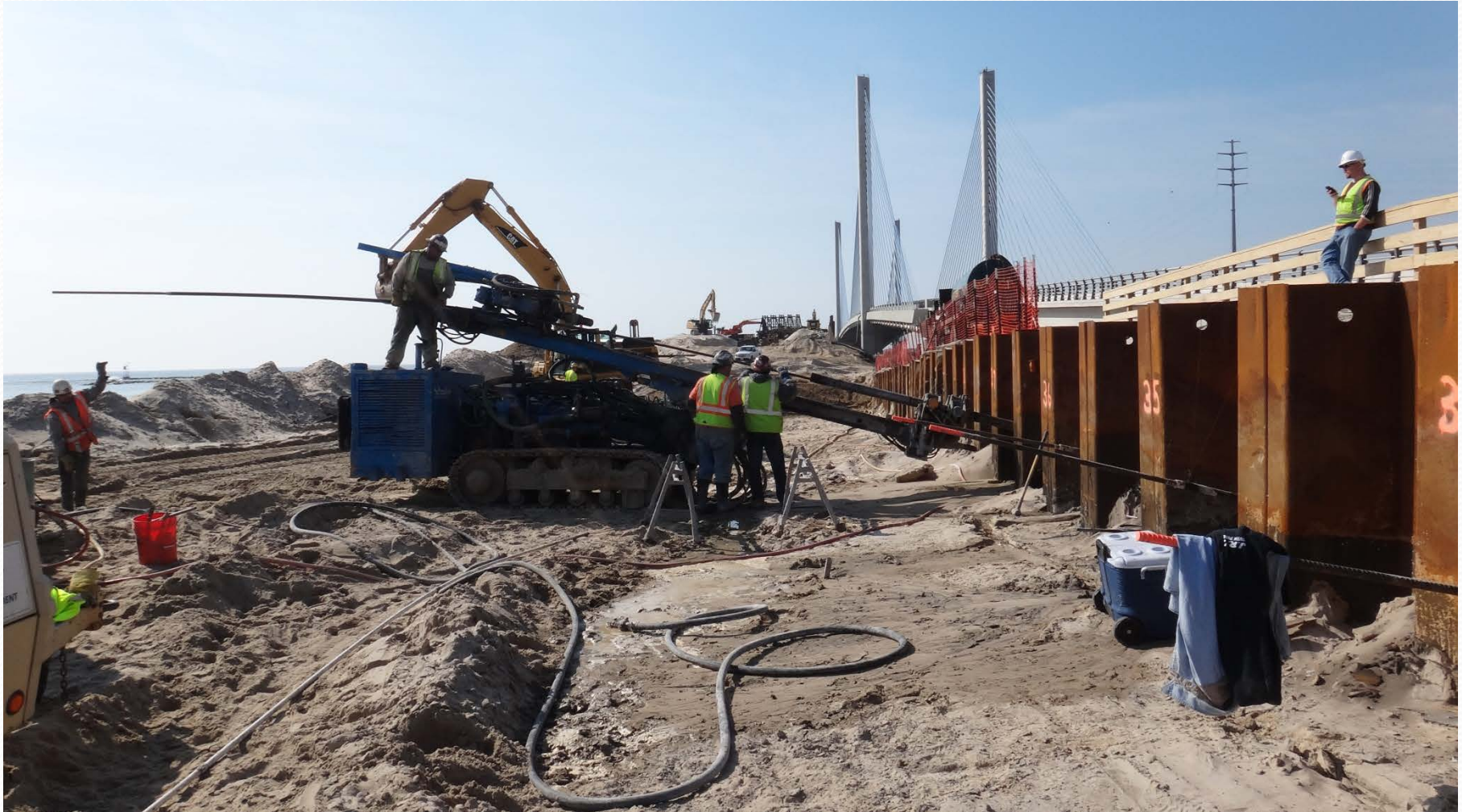
Construction of Sheet Pile Sea Wall
