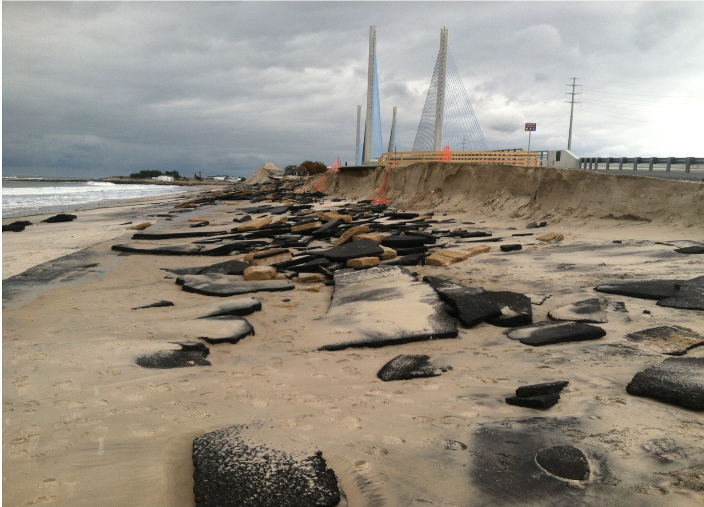
Erosion of the Approach Embankments to SR 1
