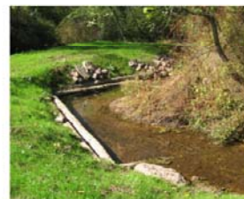
A "mud sill" protects the stream bank and provides cover for fish.
