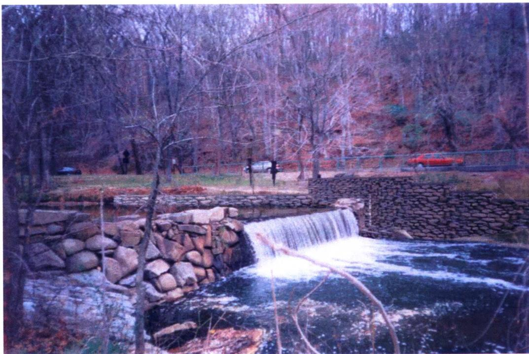
*By using similar rock to the dam itself, the fish ladder on the far bank is hardly noticeable.*
