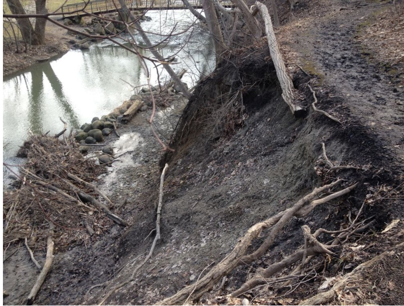
Evidence of extreme bank erosion along the shores of Pike River
