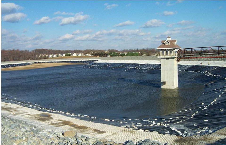
Figure A1. Newark Reservoir filling with geomembrane, concrete, and rock liner (December 2005). The geomembrane provides a waterproof lining in the lower portion of the reservoir and the concrete liner provides wind and erosion control in the upper portion of the reservoir.
