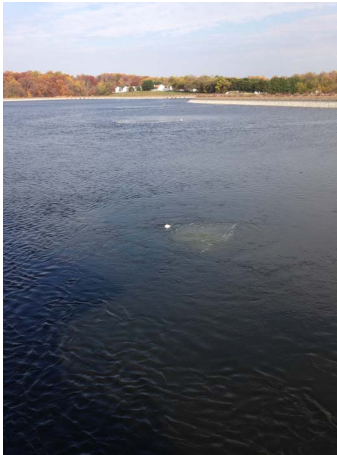
Figure A2. Newark Reservoir aeration facility installed during fall of 2016
