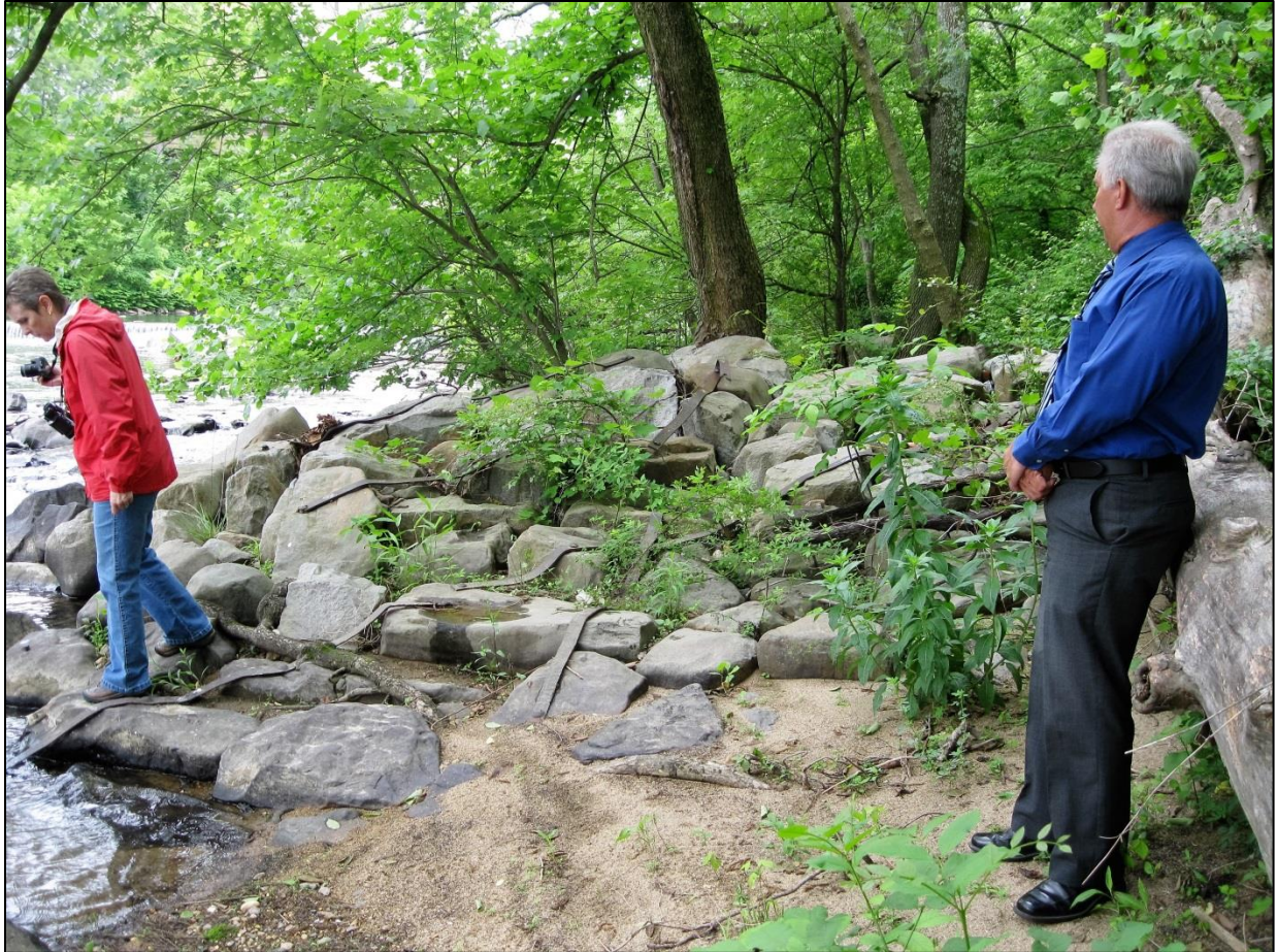
Figure 13: Historic North Bank Stabilization in the Area of the Lower Dam
