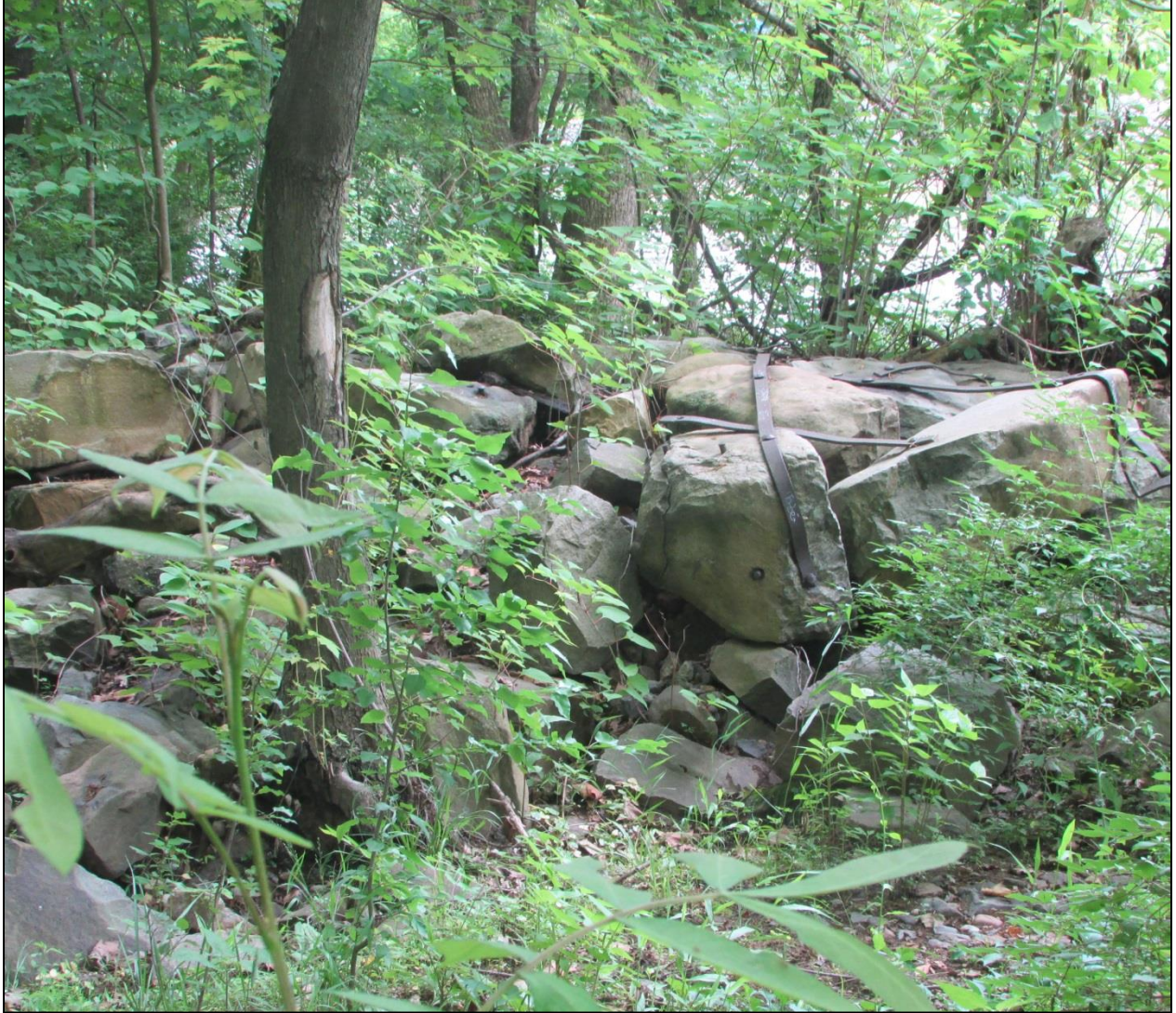
Figure 14: Iron-stabilized Masonry Wall Corner, North Bank
