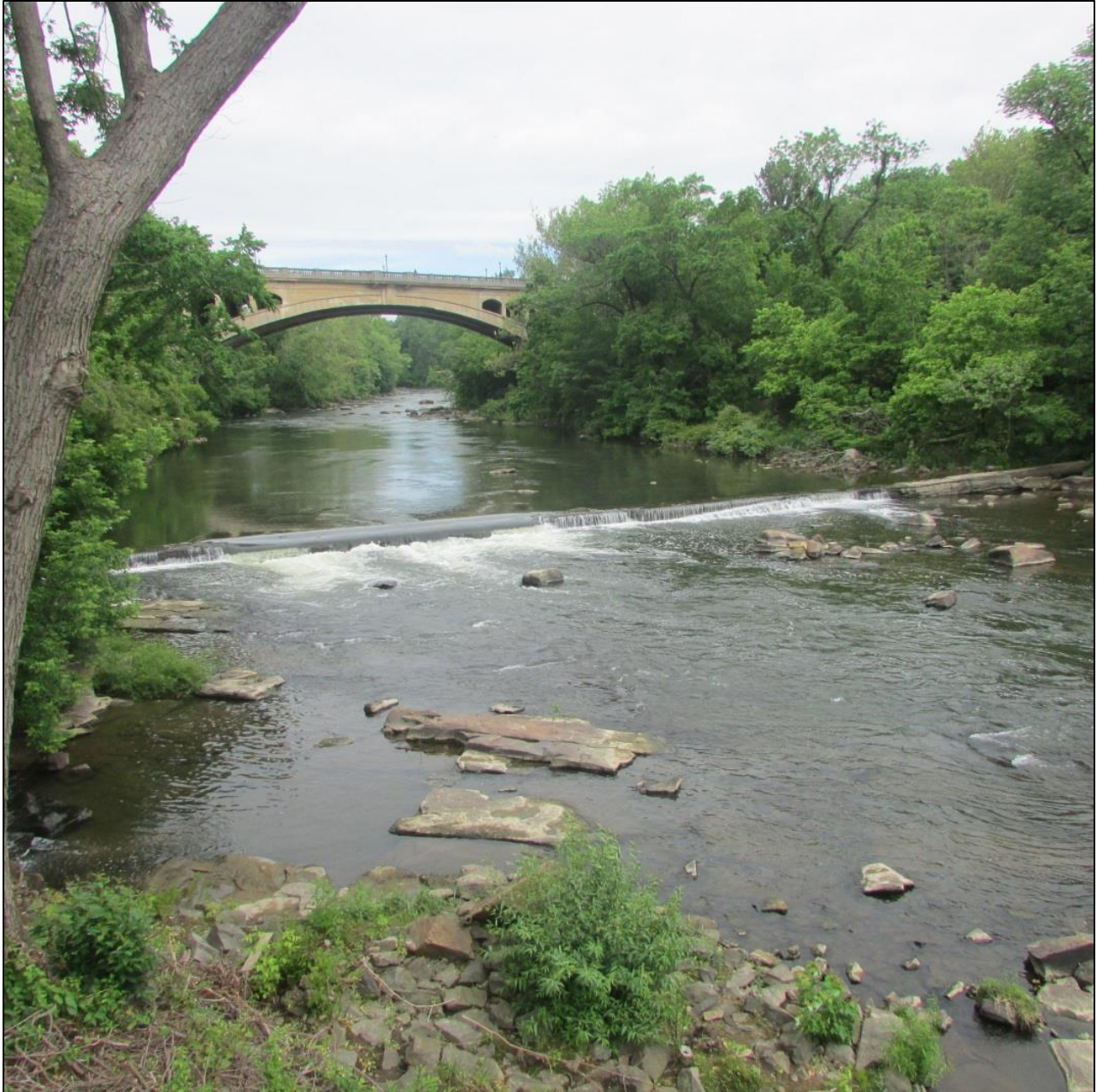
Figure 3: View of Dam 1 from South Park Drive Overlook Tower
