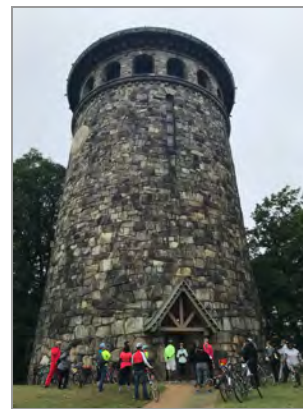
Cyclists at Rockford Tower
