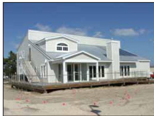
CIB's "recycled" Coast Guard barracks home, Delaware Seashore State Park, spring 2006.
