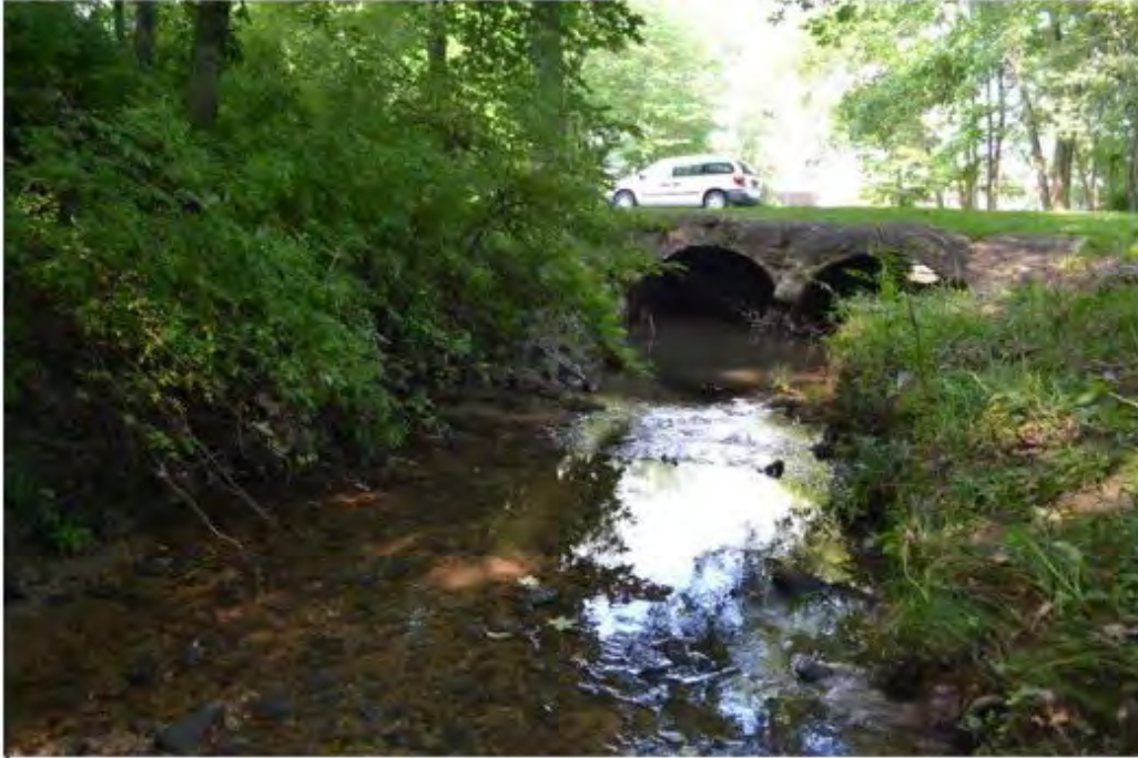
Figure 3.18. Site 12: Rocky Run Residential, July 2015 (facing downstream toward Rt. 202)
