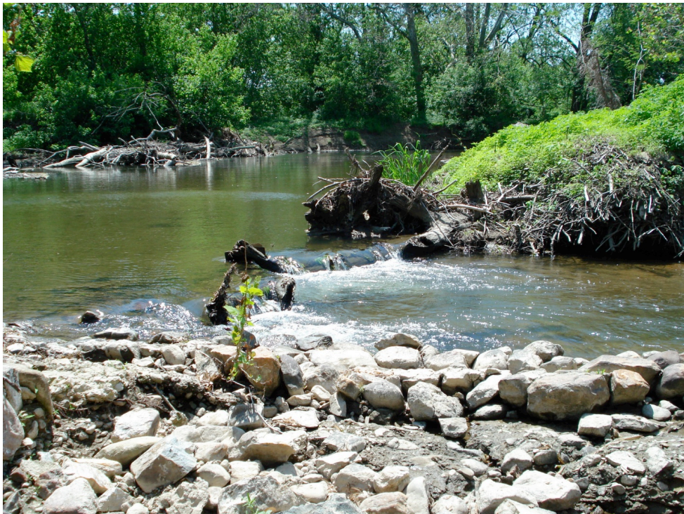
Photo 6. Dam No. 1 along White Clay Creek looking upstream at partial breach
