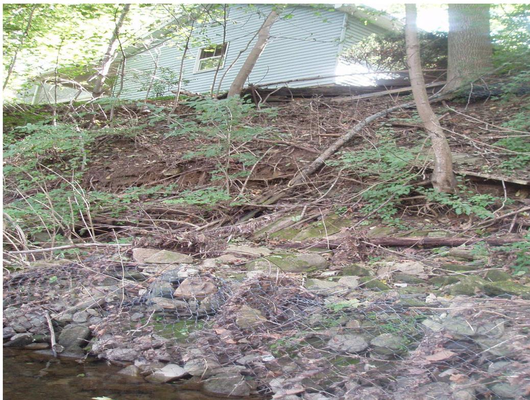
**Figure 8. Pre-restoration photo: Bank erosion along the upstream, unrestored reach near the Independence School. Gabion baskets have been installed in and attempt to stabilize the banks (Source J. Meyer 2006).**
