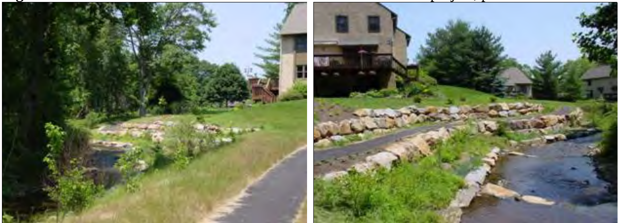
Figure 3.21. Meadowdale stream restoration and bank stabilization project, post-restoration.
