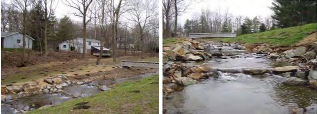
Figure 3.30. Relocated stream channel displaying a sequence of step pools.
