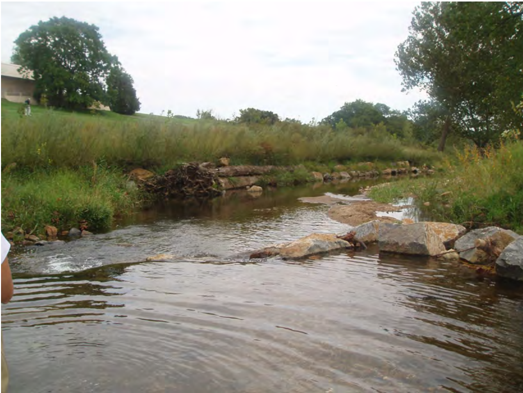
Figure 7. One year post-restoration at the Three Little Bakers Golf Course (same area depicted in Fig. 1). Log, rock and cross vanes, rootwads, and willow plantings were used to stabilize the bank, control the flow of water, and improve habitat (Source: J. Meyer 2006).
