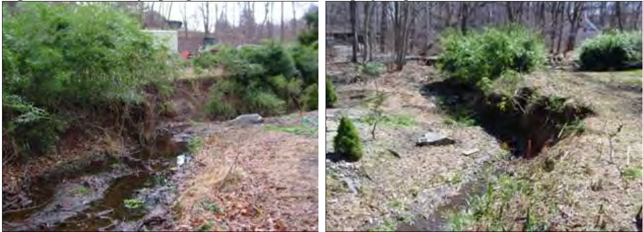
Figure 3.22. Hickory Spring road stream restoration project, pre-restoration.
