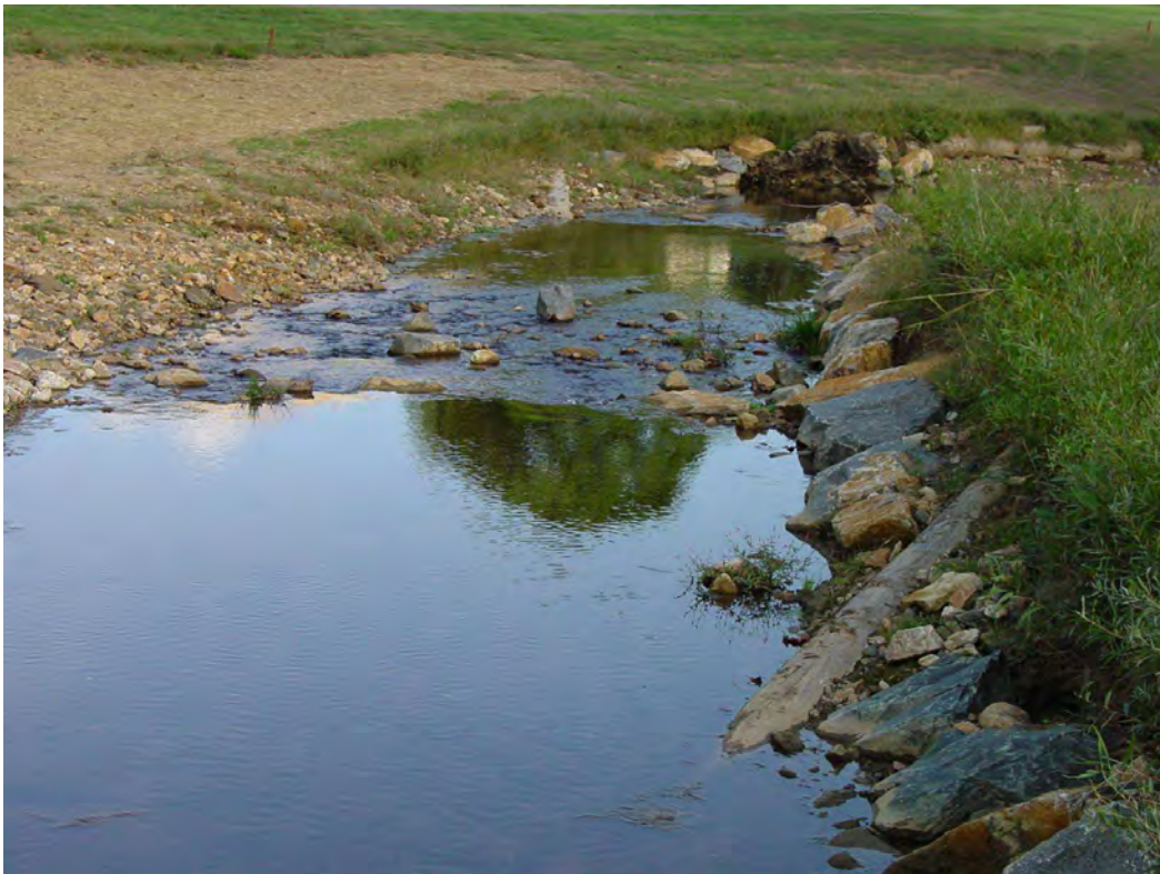
Figure 3. Post-restoration photo: Log vane (lower right corner) installed for hydrologic directional control and bank stabilization (Source: DNREC 2005).
