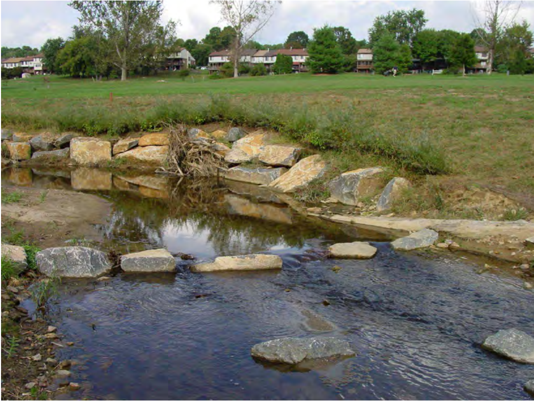
Figure 4. Post-restoration photo: Rock toe and vane, cross vane, and rootwad installed for bank stabilization, and hydrologic direction and grade control (Source: DNREC 2005).
