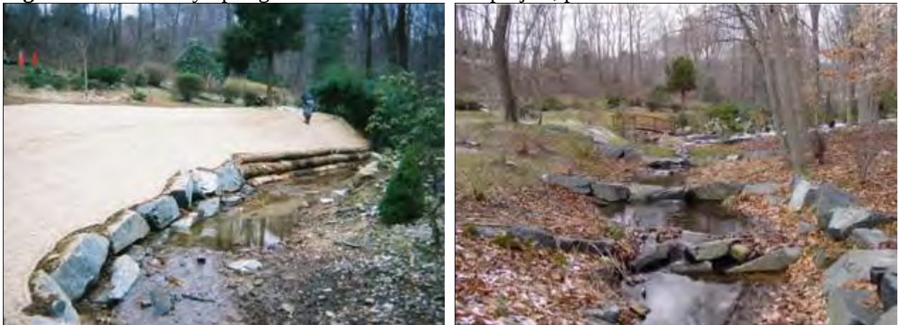
Figure 3.23. Hickory Spring road stream restoration project, post-restoration.
