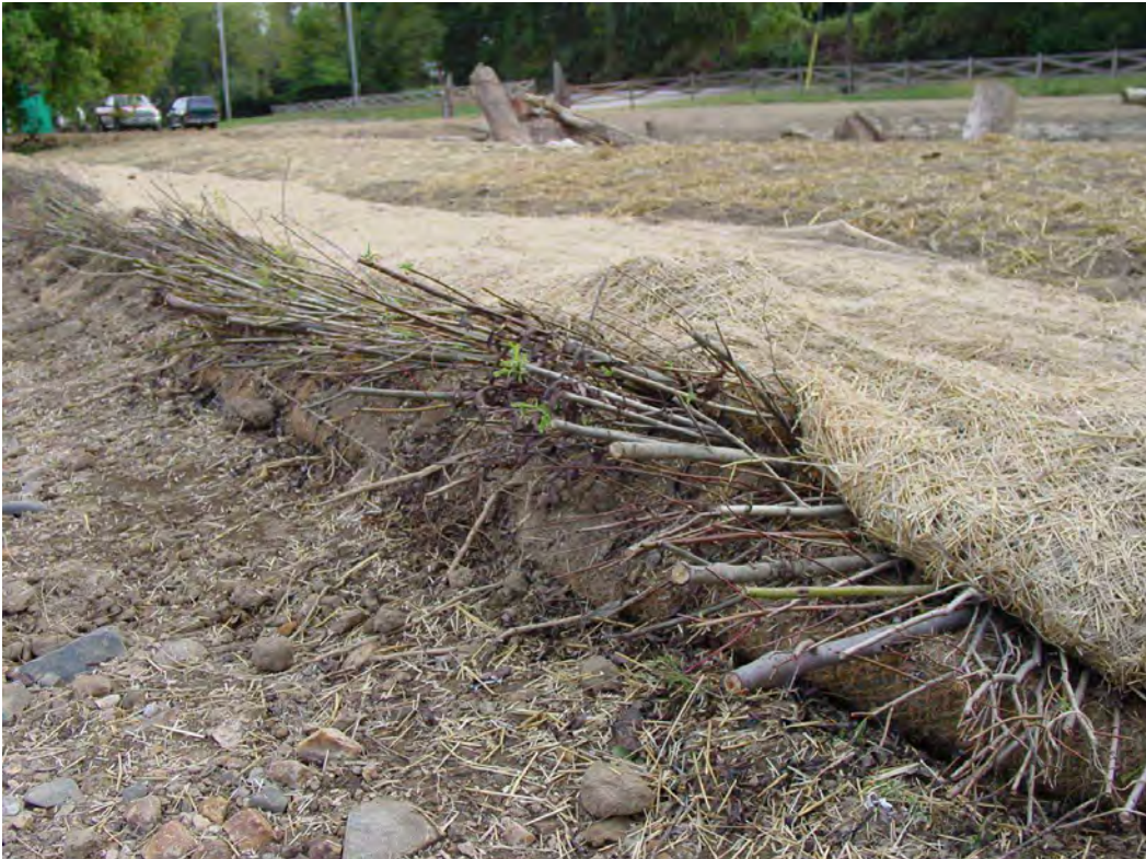
Figure 5. Post-restoration photo: Live riparian willow sprigs ( Salix sp. ) and coir matting installed for bank stabilization and to establish a riparian buffer (Source: DNREC 2005).
