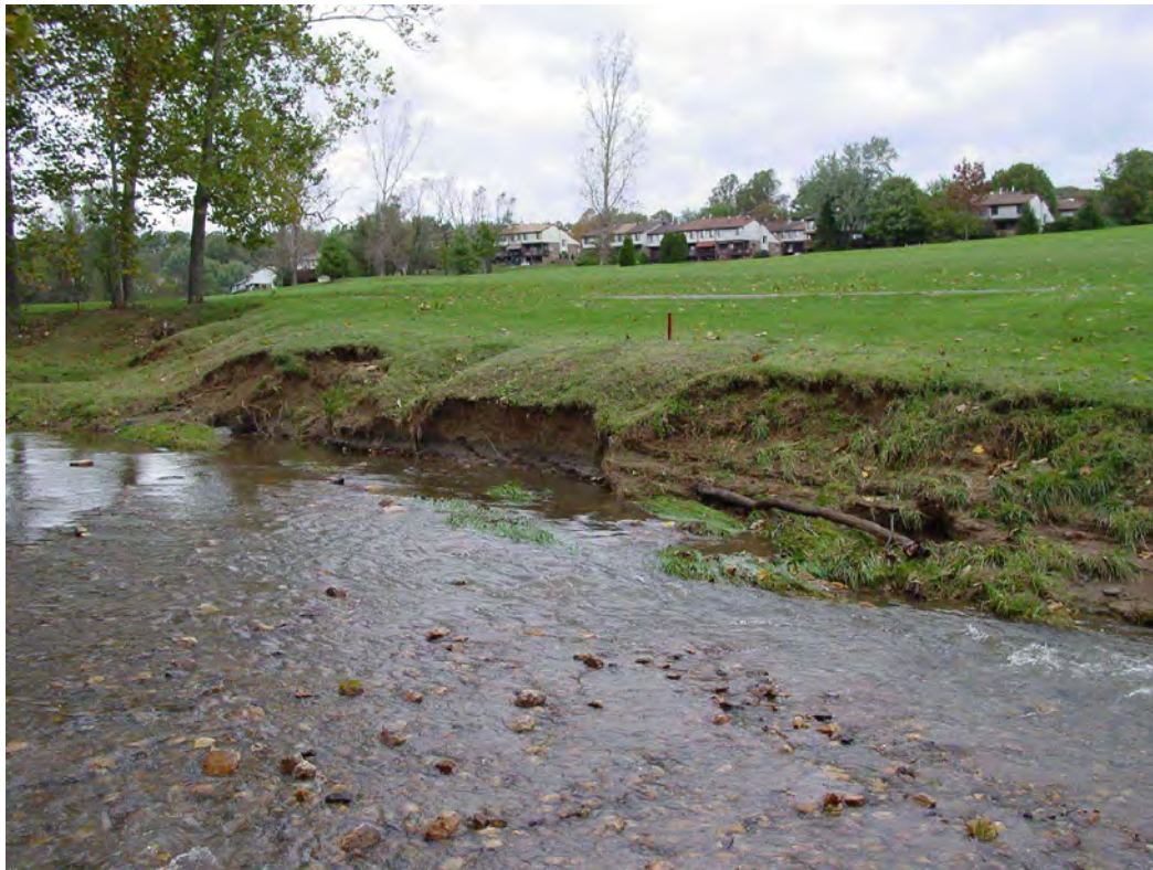
Figure 2. Pre-restoration photo: Bank erosion and slumping along Pike Creek at the Three Little Bakers Golf Course (Source: DNREC 2002).
