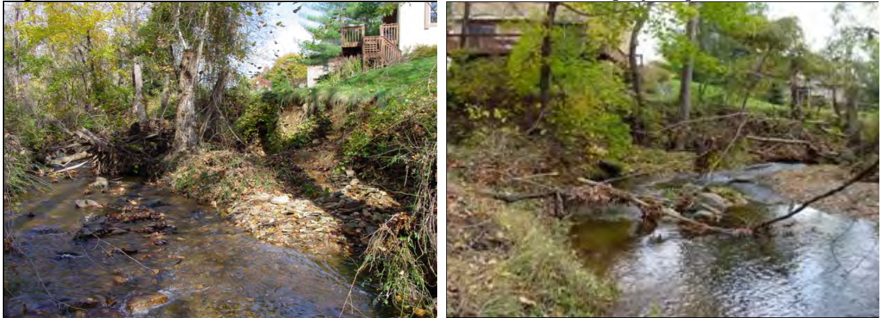
Figure 3.20. Meadowdale stream restoration and bank stabilization project, pre-restoration.
