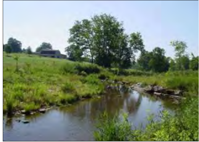
Figure 3.19. Three Little Bakers site, post-construction with stabilized stream banks.
