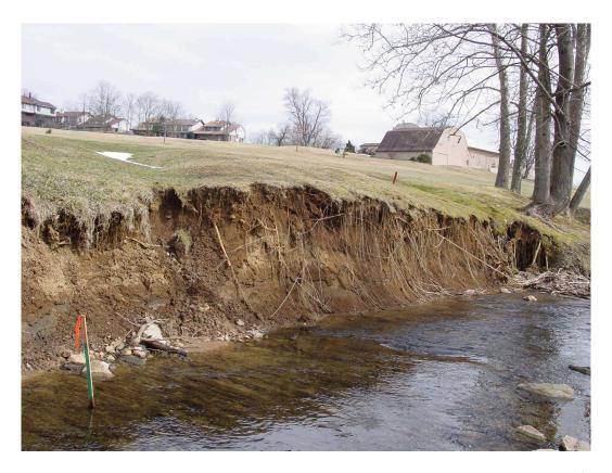
Figure 1. Pre-restoration photo: Severe bank erosion along the Pike Creek mainstem at the Three Little Bakers Golf Course (Source: DNREC 2002)
