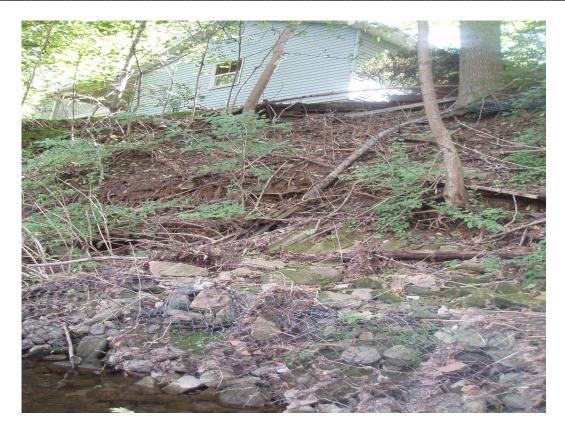
Figure 8. Pre-restoration photo: Bank erosion along the upstream, unrestored reach near the Independence School. Gabion baskets have been installed by homeowners in and attempt to stabilize the banks (Source J. Meyer 2006).
