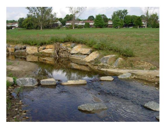
Figure 4. Post-restoration photo: Rock toe and vane, cross vane, and rootwad installed for bank stabilization, and hydrologic direction and grade control (Source: DNREC 2005).
