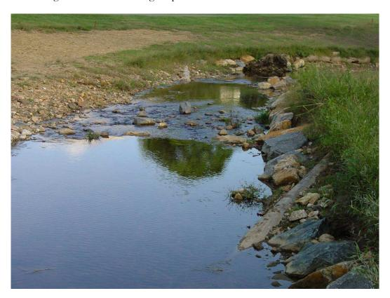
Figure 3. Post-restoration photo: Log vane (lower right corner) installed for hydrologic directional control and bank stabilization (Source: DNREC 2005).
