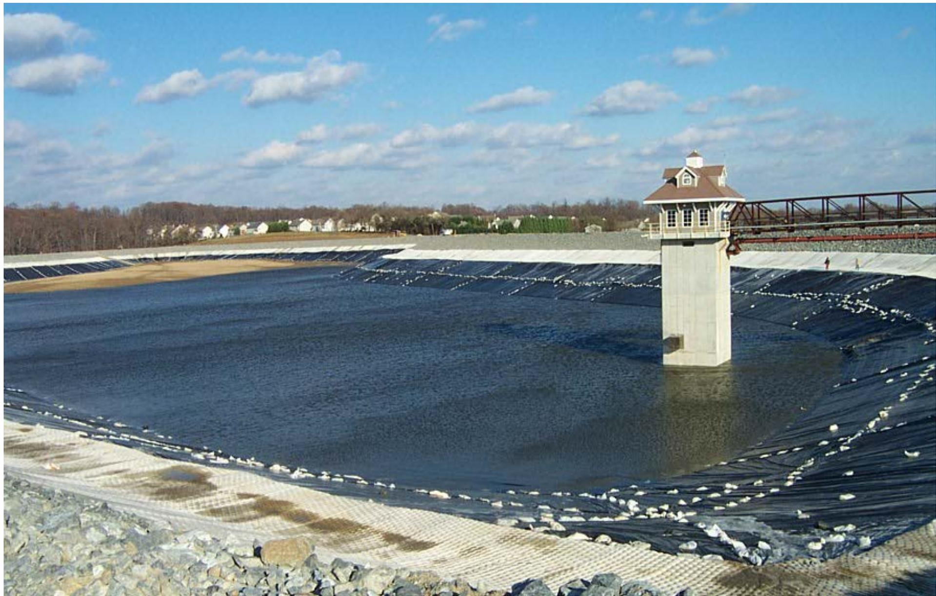
Newark Reservoir filling with geomembrane, concrete, and rock liner system
