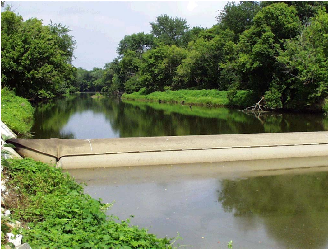
Figure 5. United Water Delaware Tidal Capture Structure (TCS).
