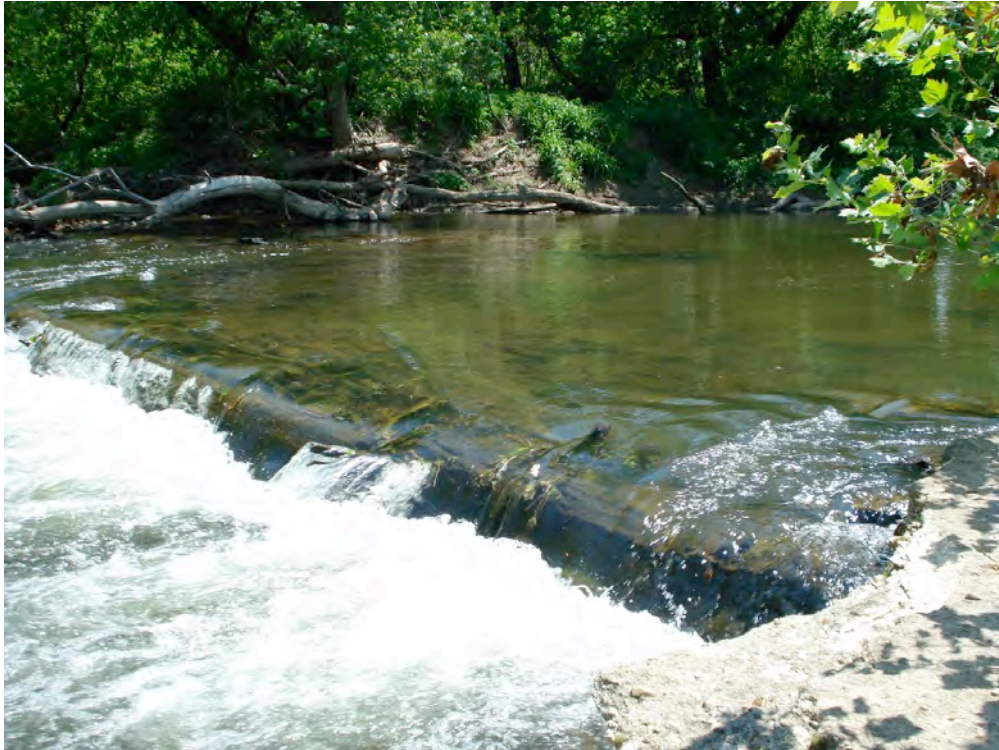
Photo 5. Dam No. 1 along White Clay Creek (RM 4.2) at Delaware Park, note timber frame
