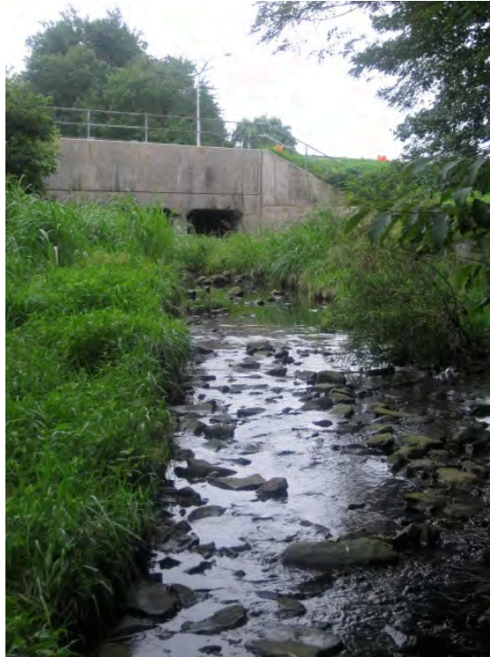
Figure 3.2. Route 202 overpass along Rocky Run
