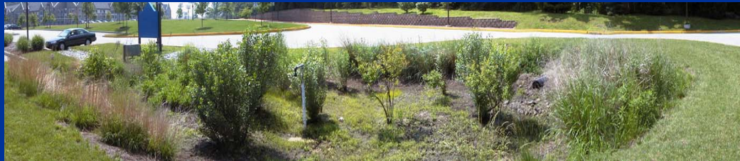
Bioinfiltration Traffic Island
