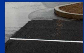
Porous Asphalt
