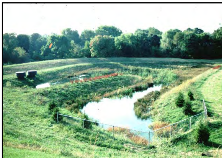
Figure 1: This shallow wetland was designed with extended detention. (Rolling Stone retrofit, Montgomery County, MD)
