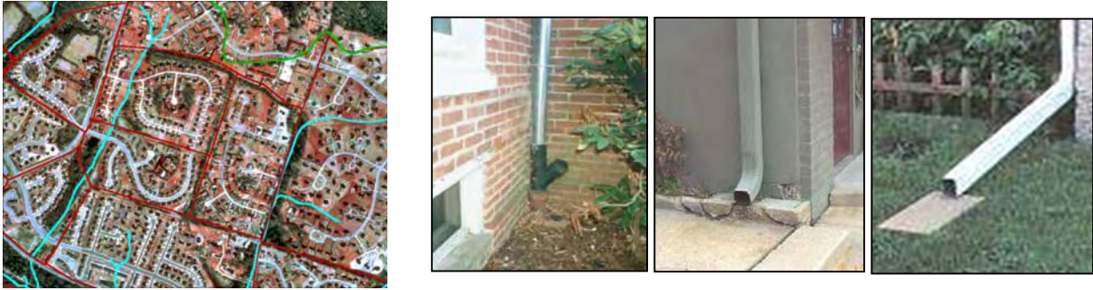
Figure 6: The Neighborhood Source Assessment (NSA) of the USSR is a useful method to determine the extent of downspout connections in a neighborhood.
