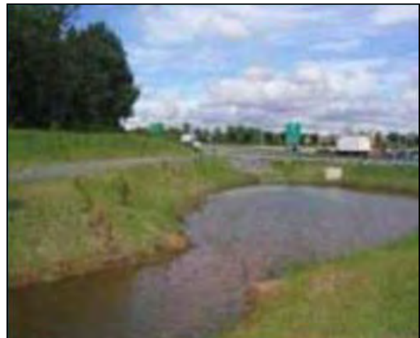
Figure 10: Retrofitting can improve the function of this failed highway practice.
