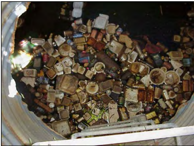
Figure 5: Routine parking lot sweeping can reduce litter collection in storm drains.
