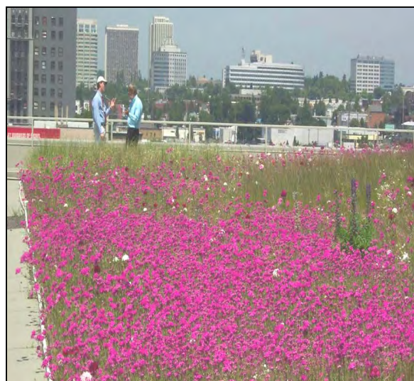
Figure 4: Green rooftops can also treat the quality of runoff from flat rooftops.
