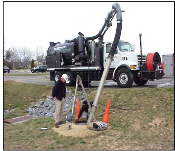
Figure 6: Mechanized rather than manual sediment removal is always preferred.
