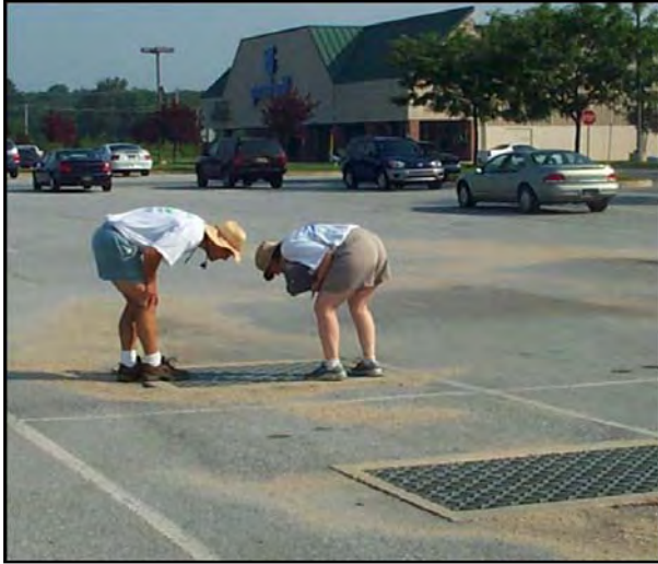
Figure 5: The crew should check out the internal plumbing of the lot to see where runoff goes.
