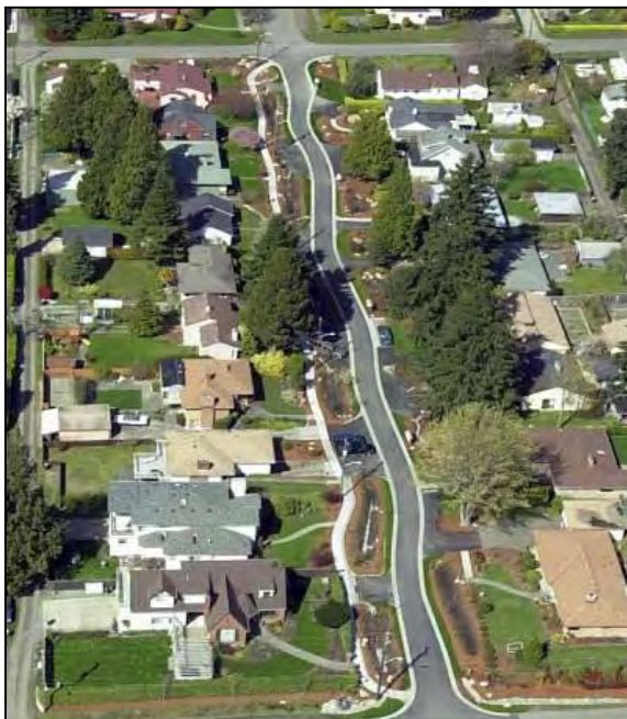
Figure 9: Aerial shot of Seattle SEA Streets retrofit.
