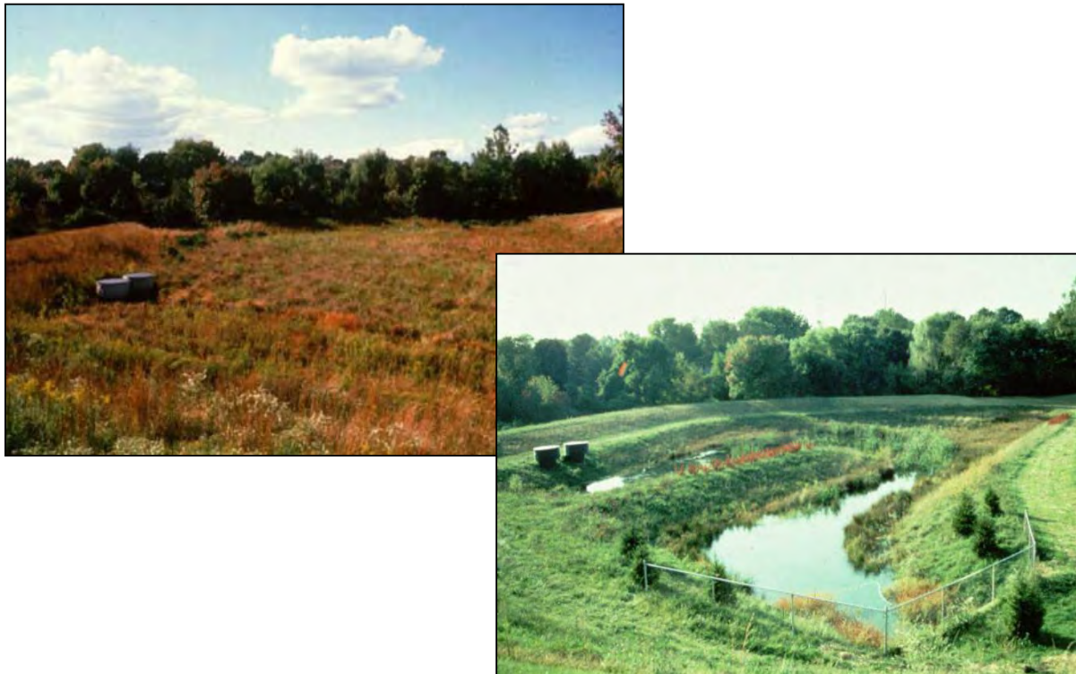
Figure 9: The Rolling Stone retrofit: before and after
