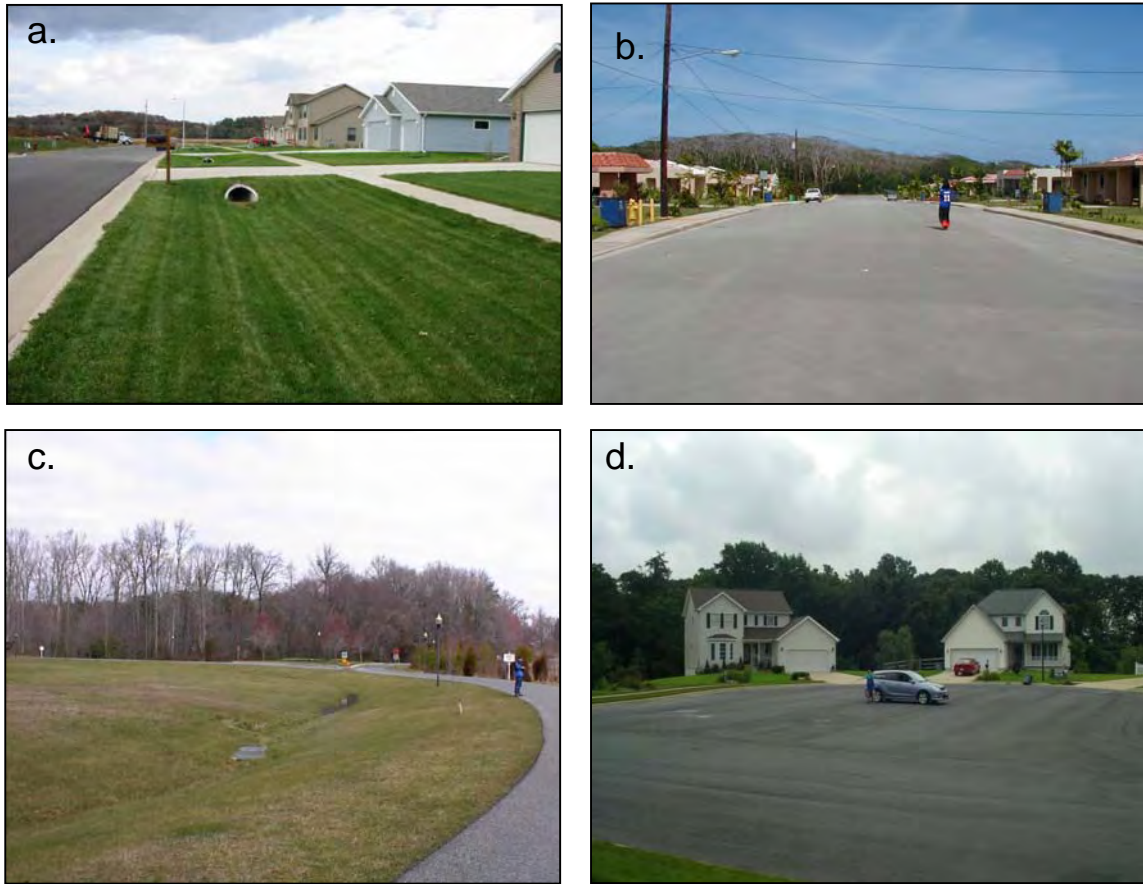
Figure 5: Ideal conditions for street retrofits include a wide right of way (a), excessively wide streets (b), open section drainage channels (c), and large cul-de-sacs (d).
