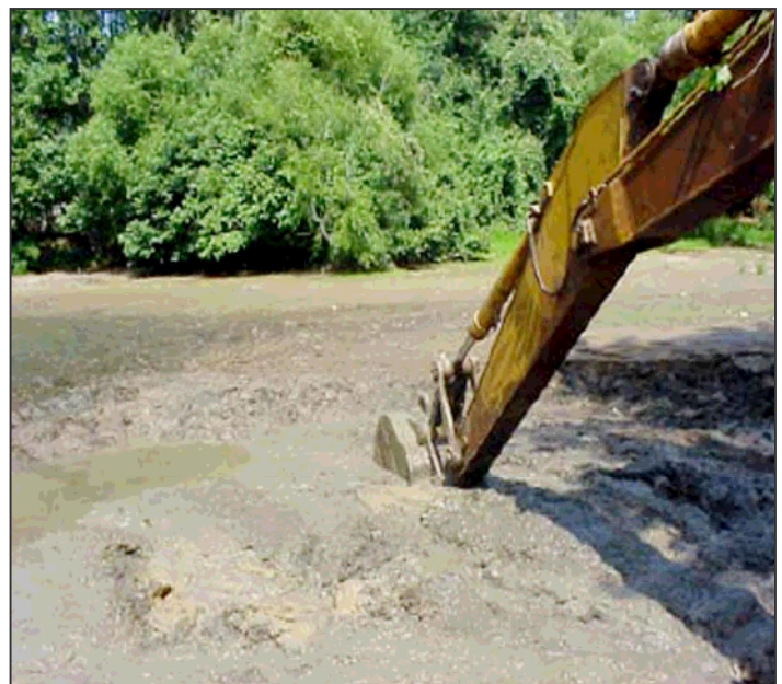
Figure 11: Dewatering is needed to excavate bottom sediments.
