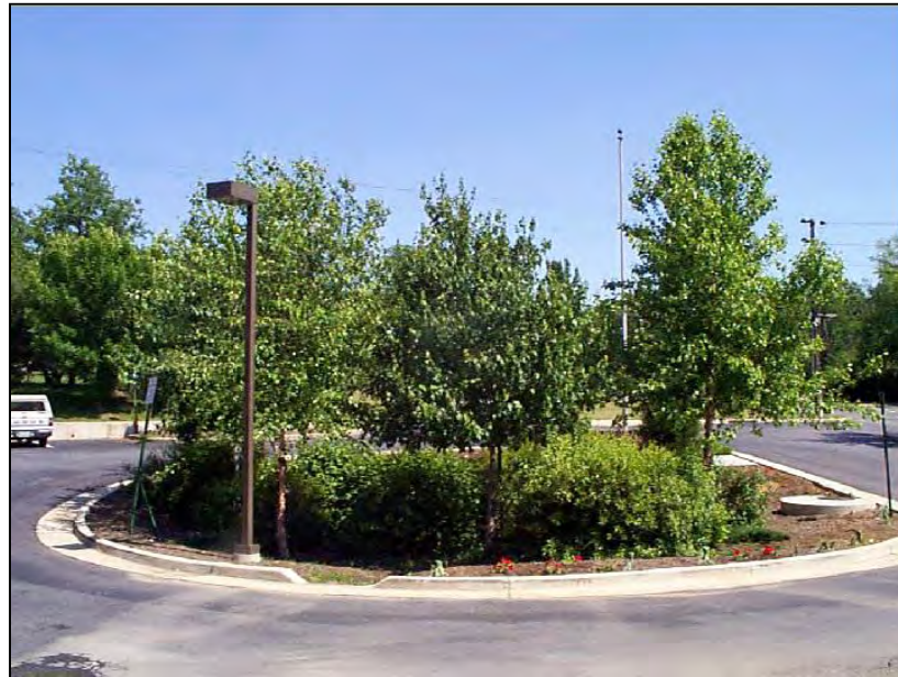
Figure 1: Bioretention created in a parking lot turn-around
