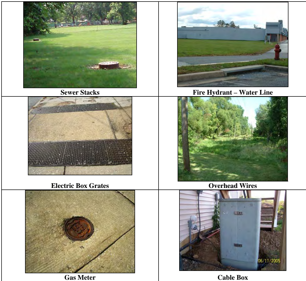
Figure 4.11: Examples of Some Common Utility Indicators
