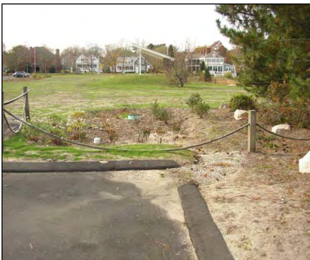
Figure 7: While ponds are most common, larger bioretention areas can provide effective treatment.
