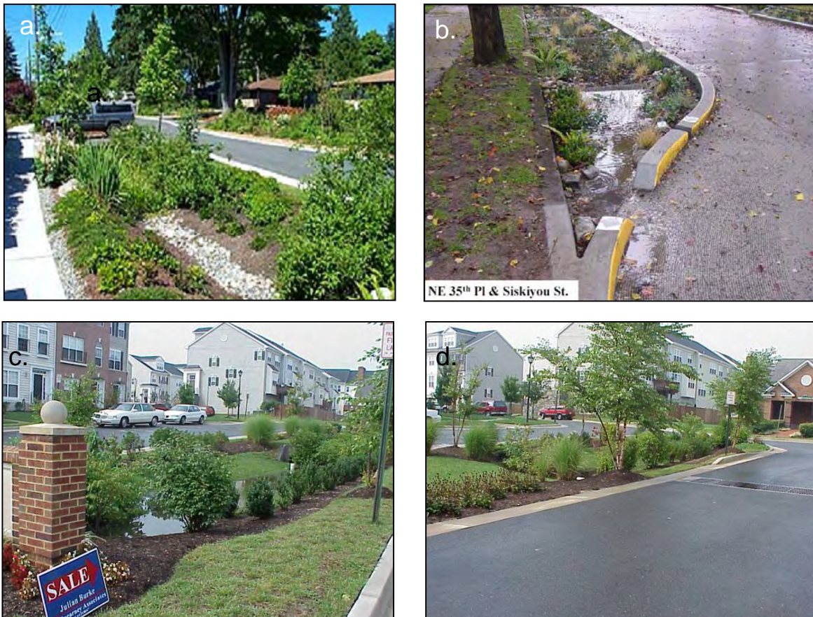
Figure 4: More street retrofit ideas: SEA streets swale (a); close-up of Portland street bioretention (b) and bioretention in street medians (c/d).
