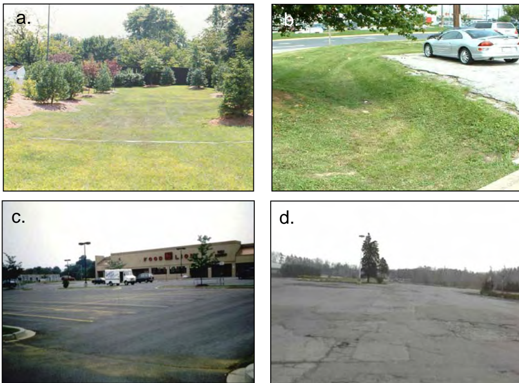
Figure 4: Ideal conditions for retrofitting small parking lots include: adjacent open land (a); unutilized setbacks along margins (b); under-utilized lots (c); and lots needing repair or rehabilitation (d).
