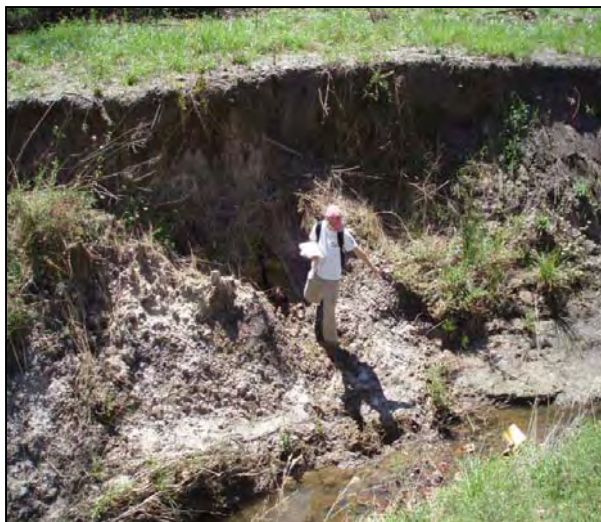
Figure 12: Designers may need to stabilize retrofit outfalls in incised urban streams.
