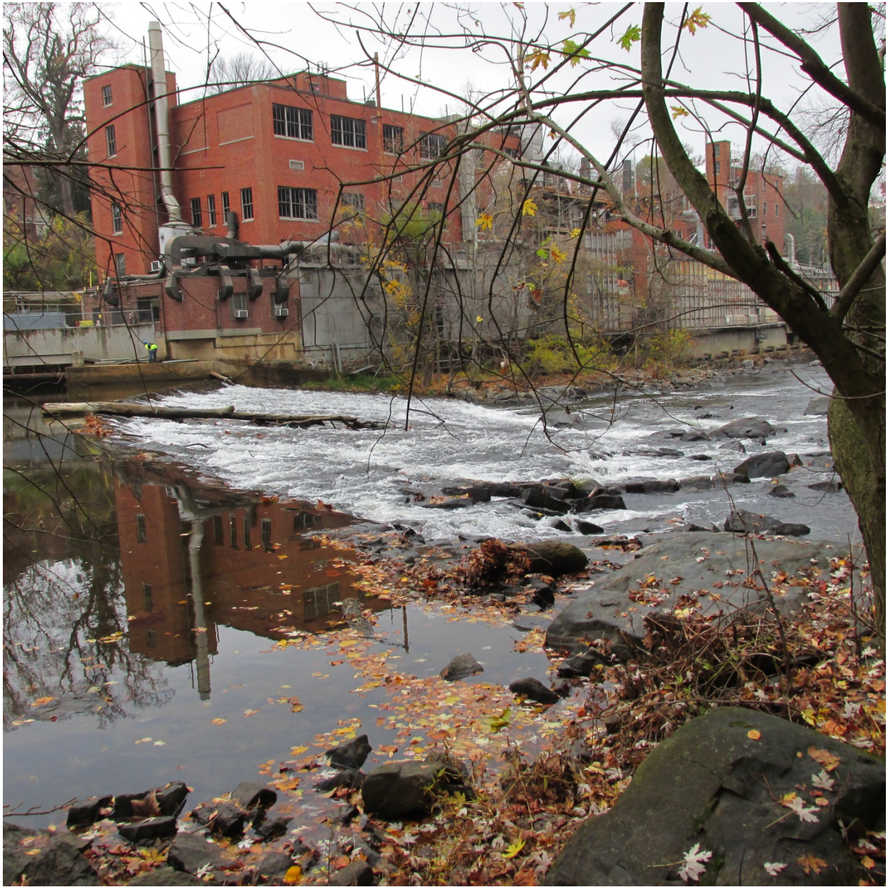
Dam 6 Looking Downstream, Partially Breeched
