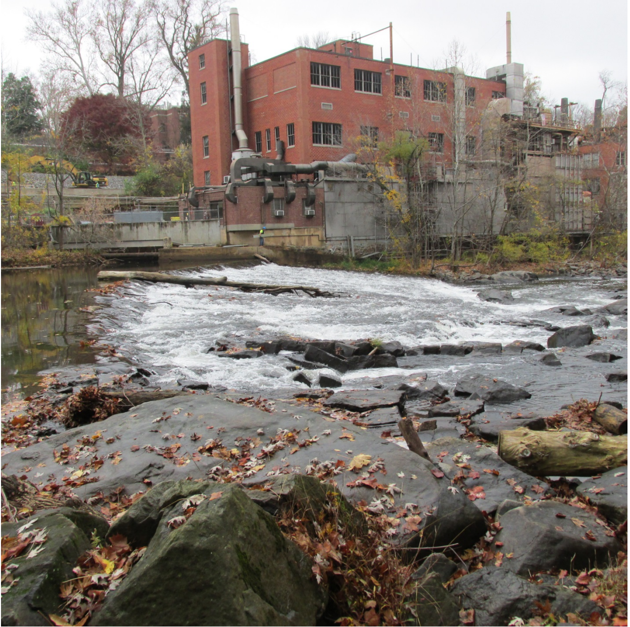
Dam 6 Looking at East Bank, Partially Breached
