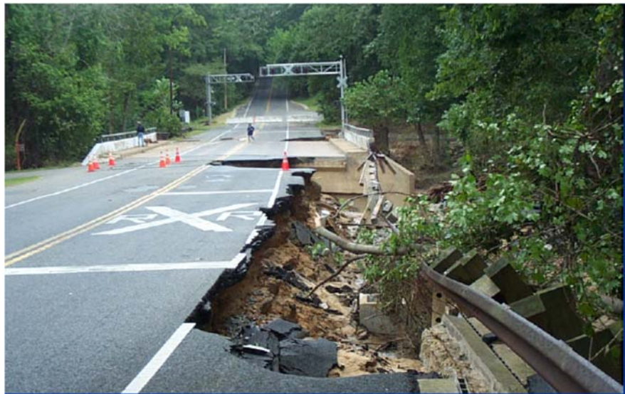
Figure 3.4. Highway damage along Red Clay Creek during September 2003 Tropical Storm Henri
