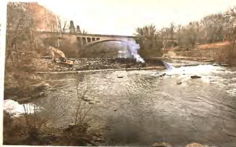
Crews are relocating a water main under Brandywine Creek as they remove a dam that has been blocking fish passage for 200 years. PHOTOS BY JENNIFER CORRETT/THE NEWS JOURNAL
