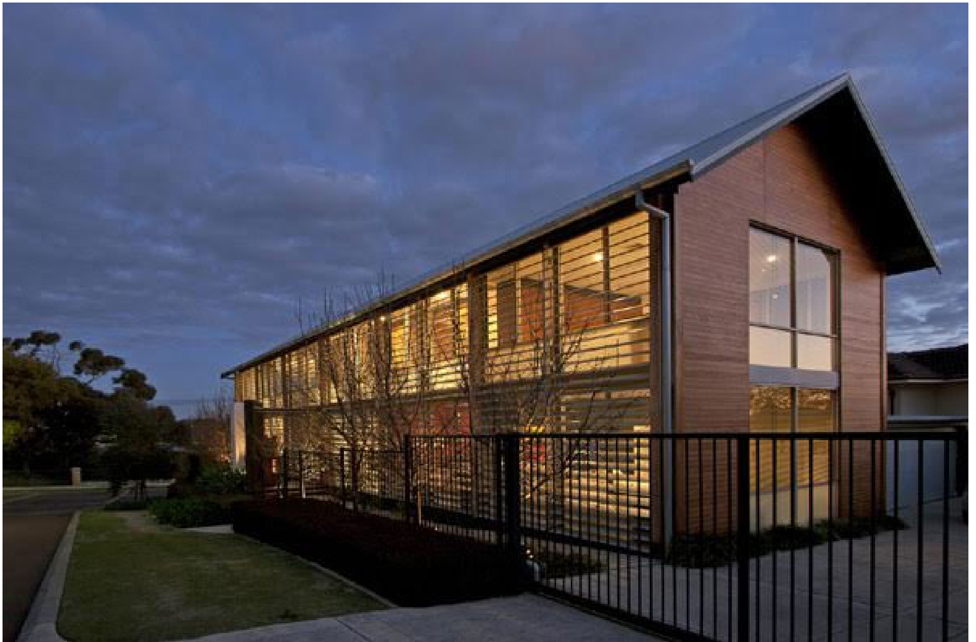
Future University of Delaware Water Resources Center Building
