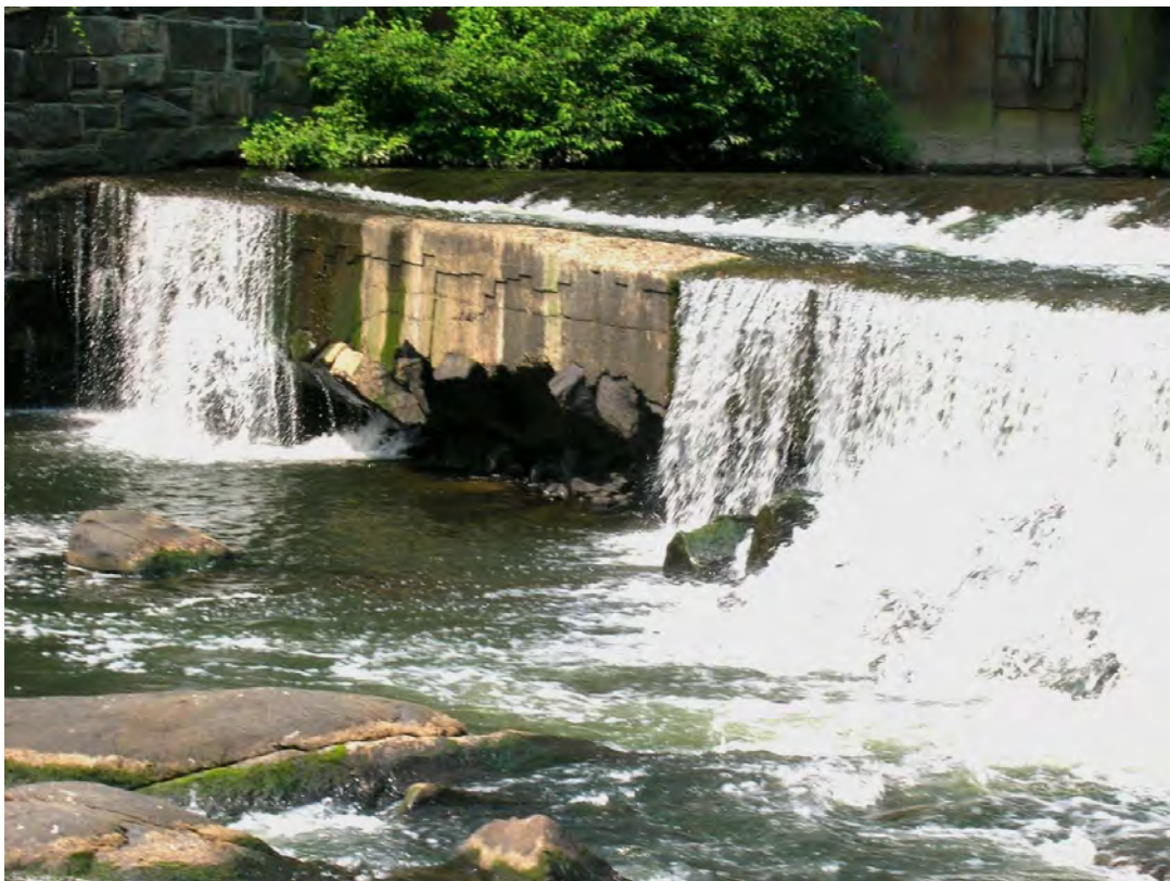
Bancroft Dam 4, damaged in center of dam
