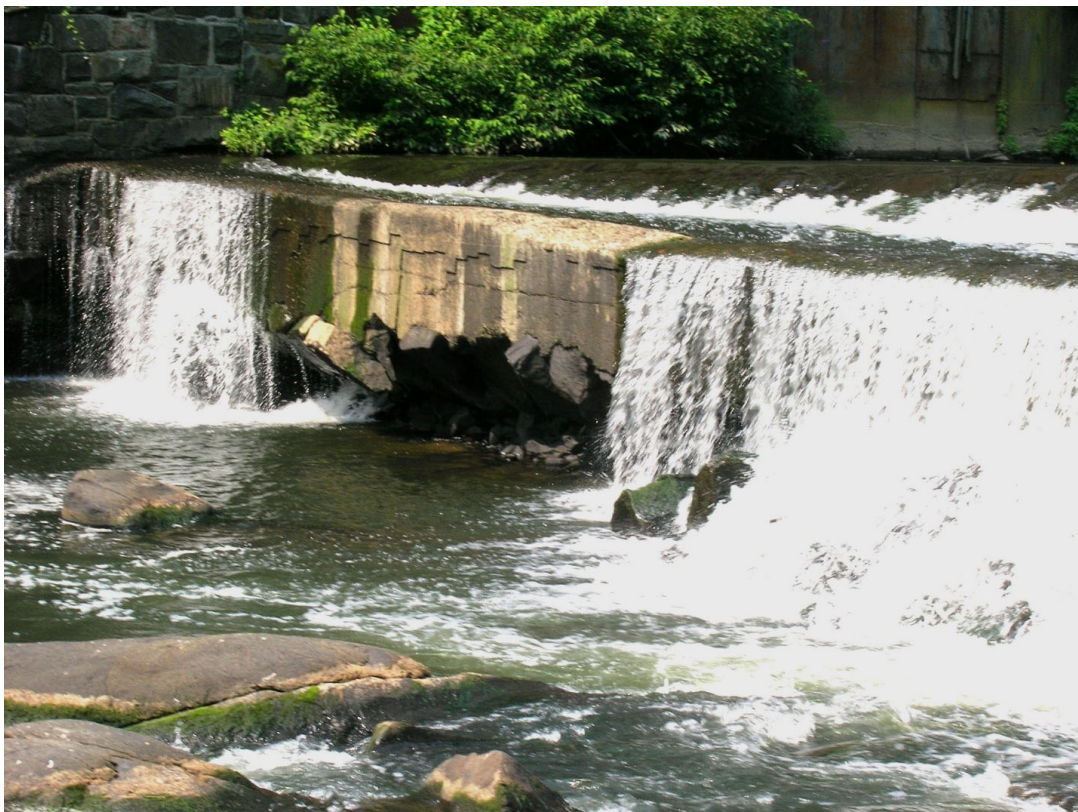
Bancroft Dam 4, damaged in center of dam
