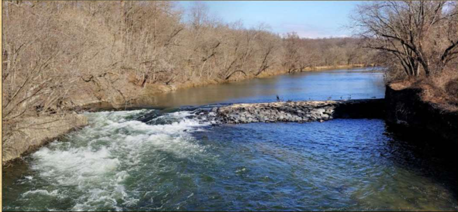
Dam: 5-foot-high, 125-ft. long, made of locally-obtained blue granite; located 200 ft. upstream of the current bridge. Later raised to 7 feet. West one-third breached c. 1999 (Floyd)
