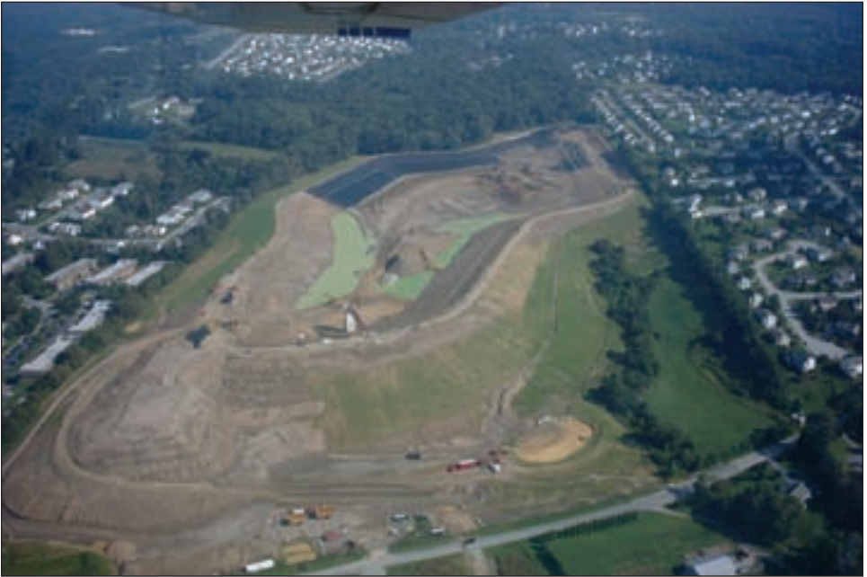
Figure 19. Newark Reservoir under construction during summer of 2004 (source: City of Newark, 2004)
