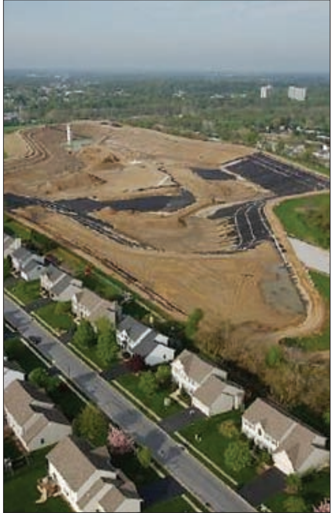
Figure 18. Newark Reservoir construction in May 2004 (source: City of Newark, 2004)
