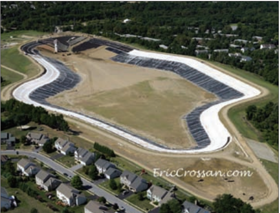
Figure 20. Newark Reservoir under construction in June 2005 (source: Eric Crossan, 2005)
