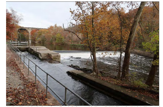
Figure 26. View of Dam 2, showing the southern mill race in the foreground, looking north, 2021. (Center for Historic Architecture and Design)
