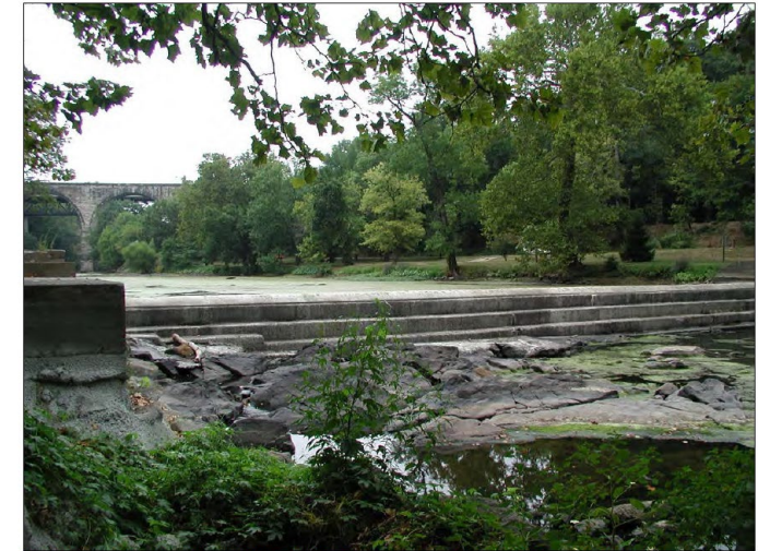
Figure 22. View of Dam 2 during low water flow, showing stepped concrete construction, looking north, 2002. (Water Resources Center, University of Delaware)
