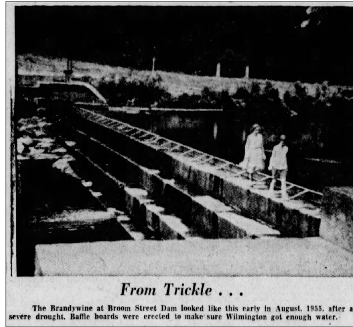
Figure 21. August 1955 view of Dam 2 showing stepped concrete construction. (Journal-Every Evening, February 7, 1959)
