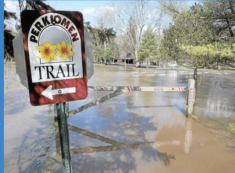
Flooding on the Perkiomen Trail from Hurricane Ida (The Times Herald, 2021).
